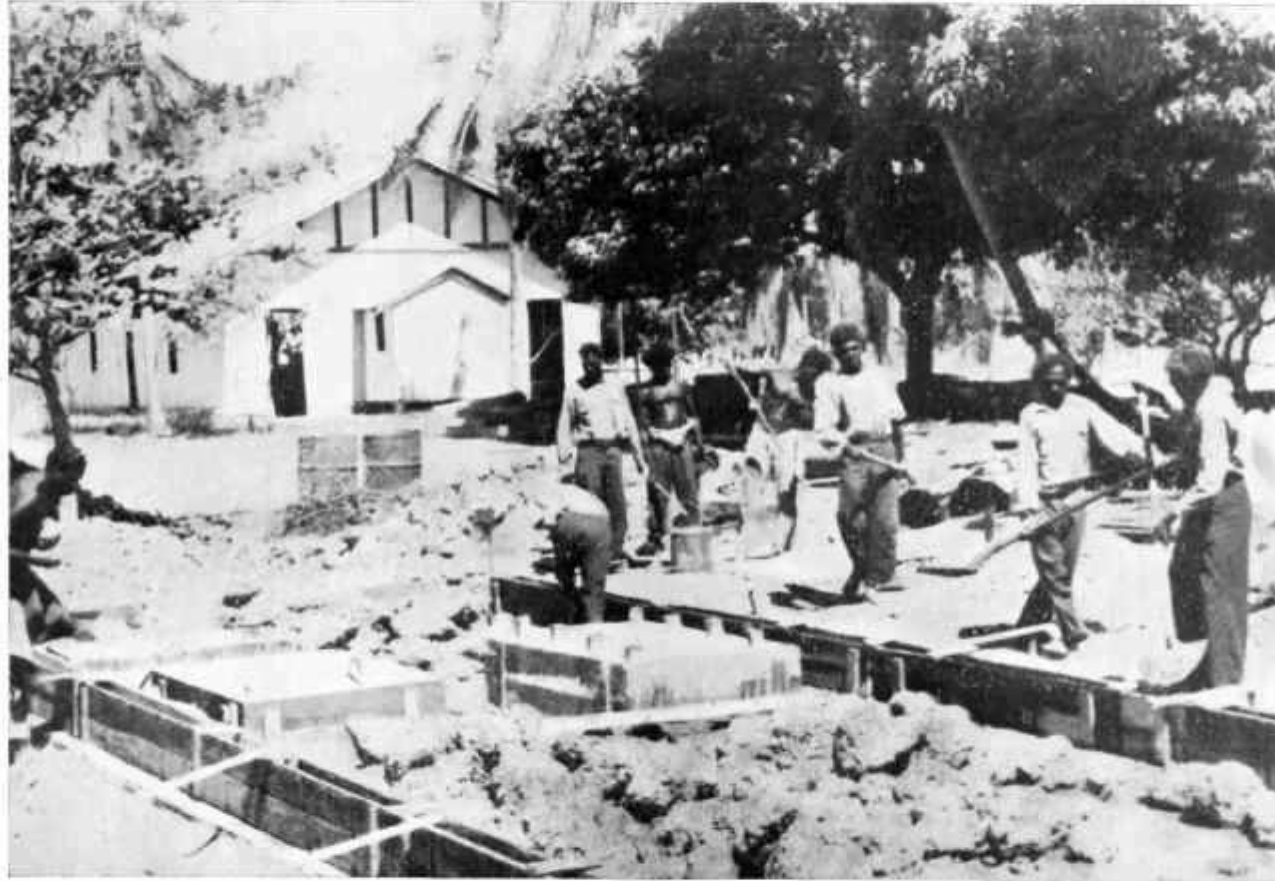
Construction of Cold Room, Aurukun Mission.
