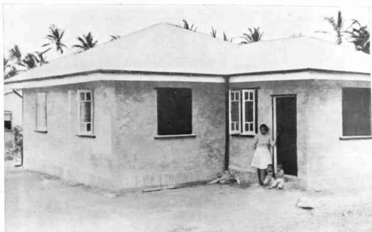
Completed Concrete Brick Native Cottage, Palm Island.
