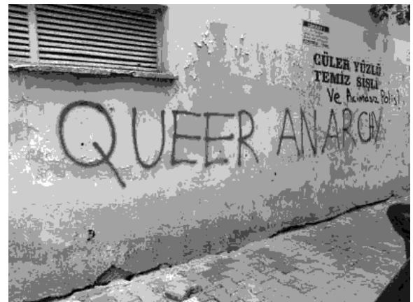
Windows broken, slogans painted at Haliç University in Istanbul, Turkey, 01.05.14
