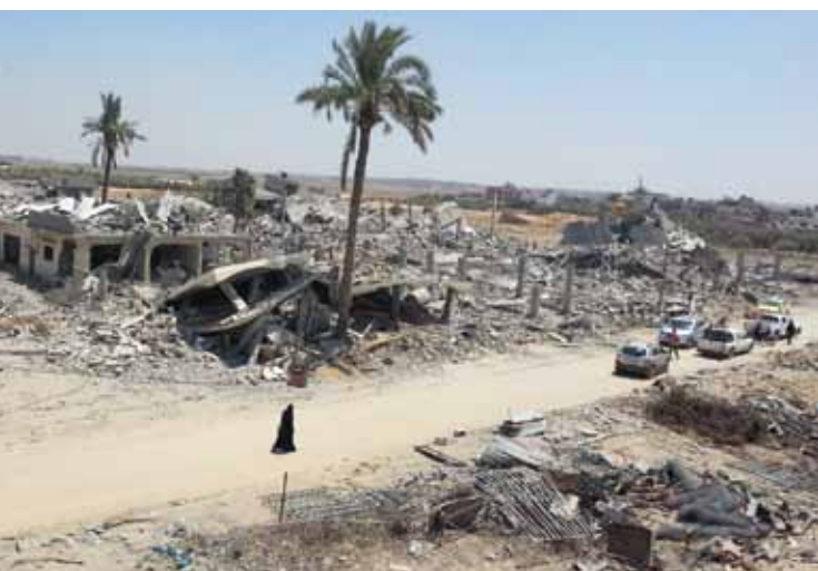
Part of the destruction left in Khuza'a village east of Khan Yunis
