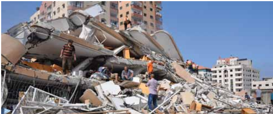
Remnants of al-Zafer (4) multi-storey building that was destroyed by Israeli forces in Gaza City
