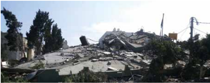
Remnants of the Financial and Administrative Monitoring building, west of Gaza City
