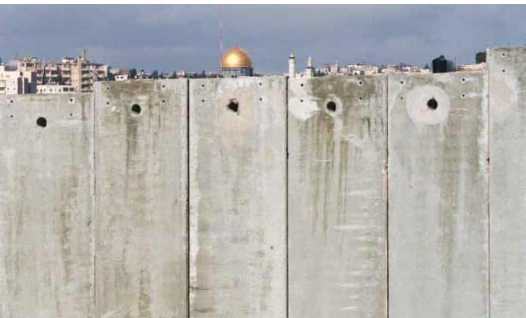
The annexation wall in the oPt
