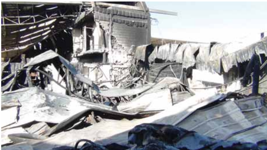
Part of destruction in al-Srou factory
