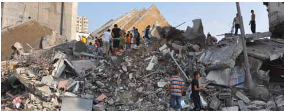
Remnants of al-Basha multi-storey building that was destroyed by Israeli forces in Gaza City
