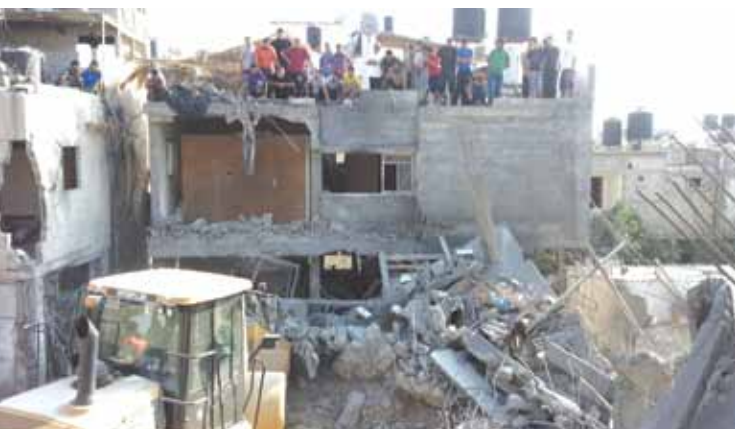
The remnants of the al-Batash family's house in al-Tuffah neighborhood in the east of Gaza City
