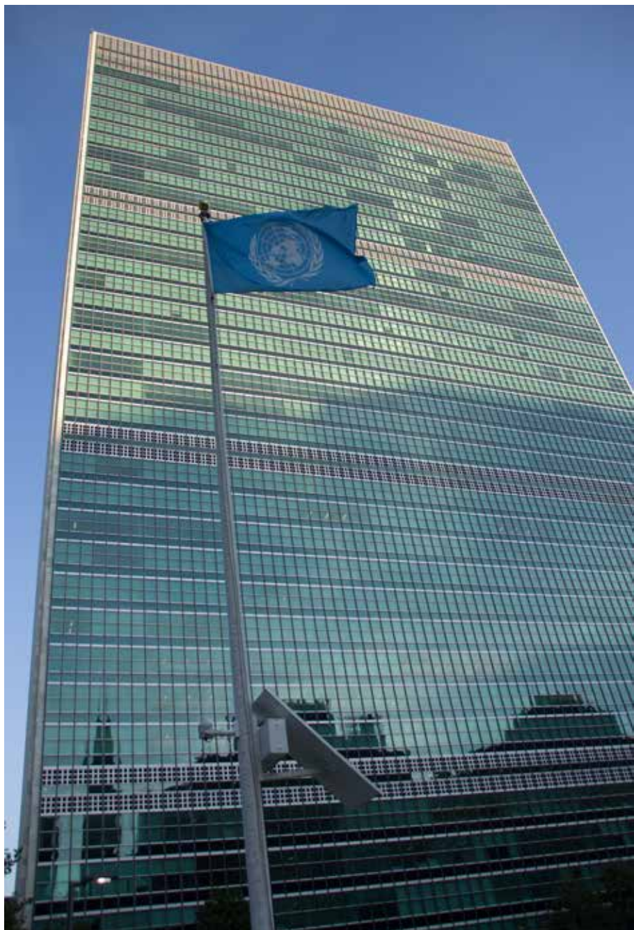
A close-up of east-facing windows on the United Nations Headquarters Secretariat building in New York. ■ UN Photo/KELVYN PEREZ
