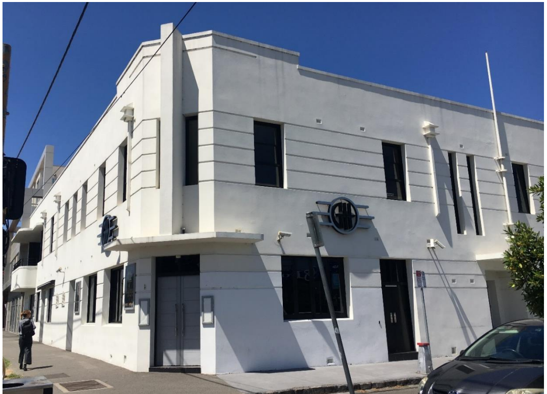
Figure 8. Current view of the Greyhound Hotel showing the corner orientation. (Context, 2017)
