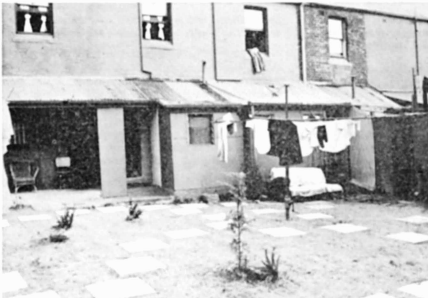
This photo shows the state of the backyards after temporary renovations and work on the project
