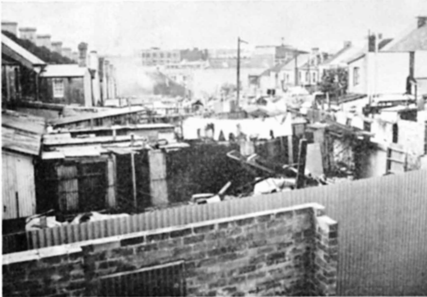
This photo shows the state of the backyards of the homes prior to work on the project
