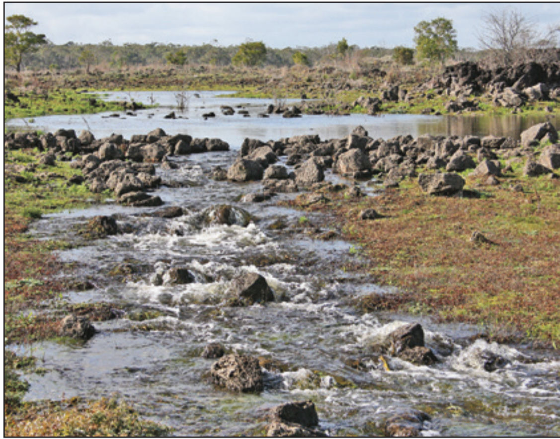
Budj Bim in south-west Victoria is the world's oldest remaining engineering project, and Gunditjmara traditional owners are seeking UNESCO World Heritage listing for the site.
