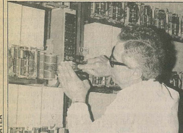
Step by Step exchange: first introduced in 1915. For an average telephone exchange of 10 000 lines, 15 people would be employed.
