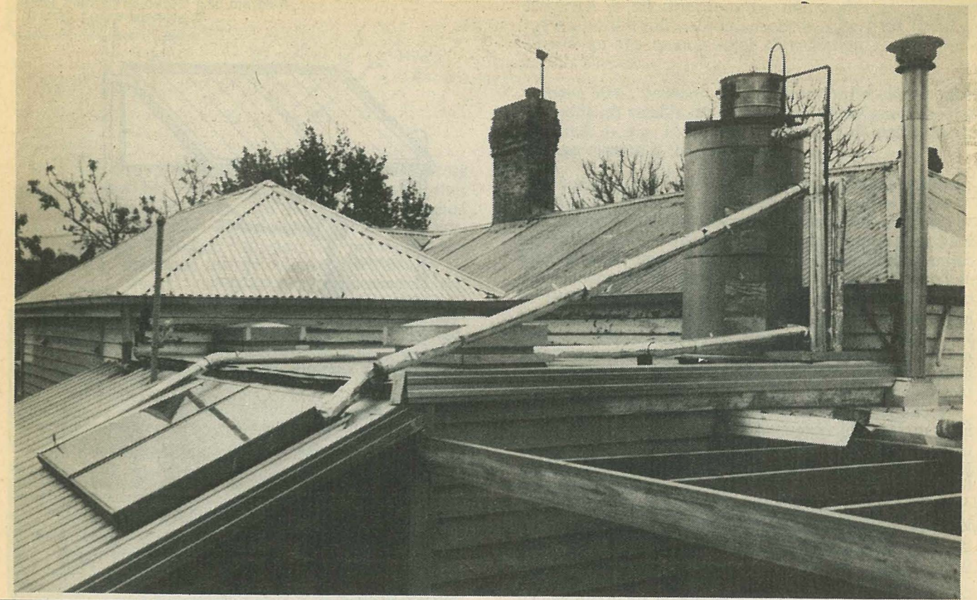
A solar hot-water system tucked away at the back of a house in Surrey Hills, Melbourne.
