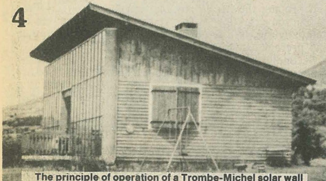
The principle of operation of a Trombe-Michel solar wall and a house at Odeillo, France, which uses this system to supply 60-70 per cent of the annual energy needed for space heating.
