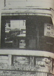
Members of the National Union of Railworkers have been pressing for twelve months for repairs and maintenance work at Bowral and neighbouring towns.
