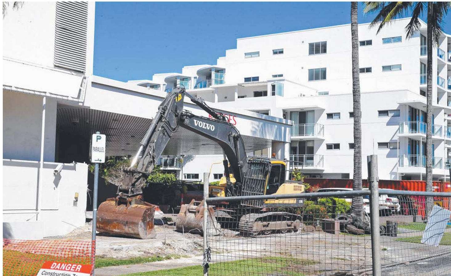
Heavy machinery at the former Rydges Tradewinds which is being renovated.
