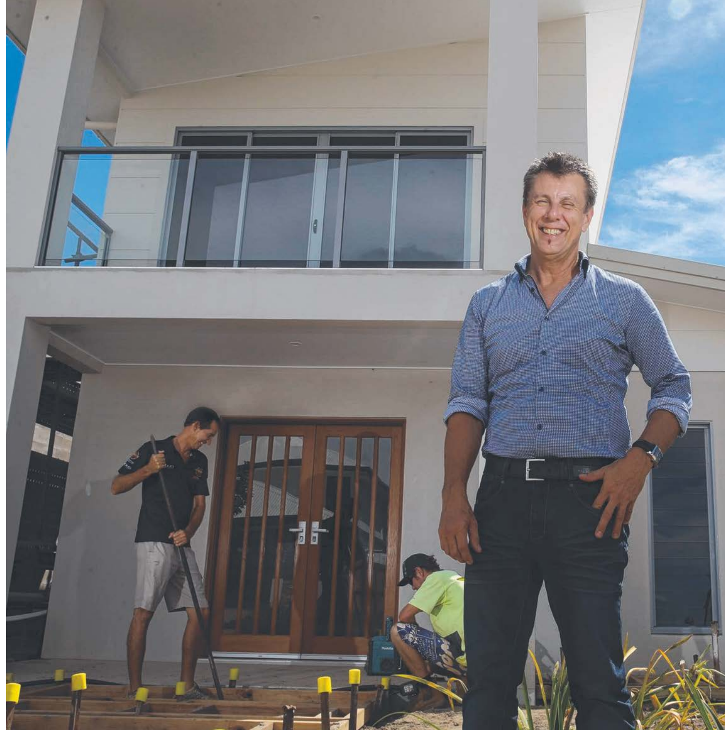
HIA Cairns branch manager Russell Parnicott at a house under construction at Trinity Beach
