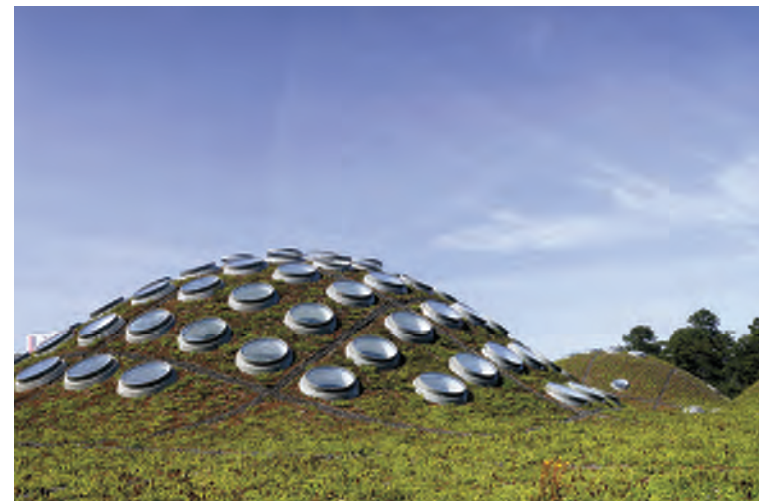
CALIFORNIA ACADEMY OF SCIENCE, SAN FRANCISCO, RENZO PIANO BUILDING WORKSHOP, 2008
