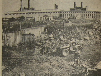
The foundations for Newport. That's all there's been for years, though completion was set for 1972. The old powerhouse is in the background.
