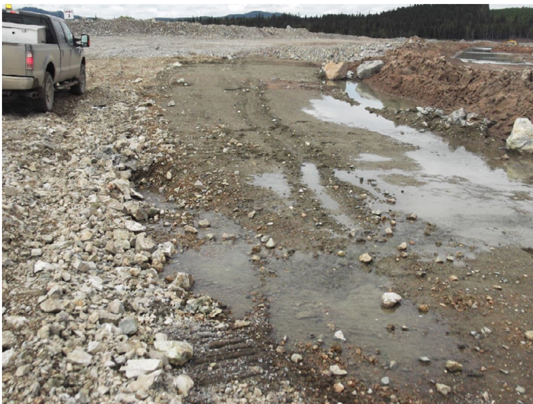
Figure 6.25 Water Overtopping Embankment Core and Entering Filter Zone, Station 1+530 on SE, May 24, 2014 AMEC (2014d) p. 5
