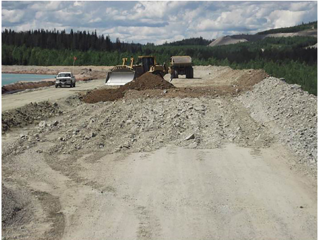
Figure 4.3 Placement of Zone C Rock near the area of the breach, June 26, 2014, Mount Poilley Mining Corporation (2014c)
