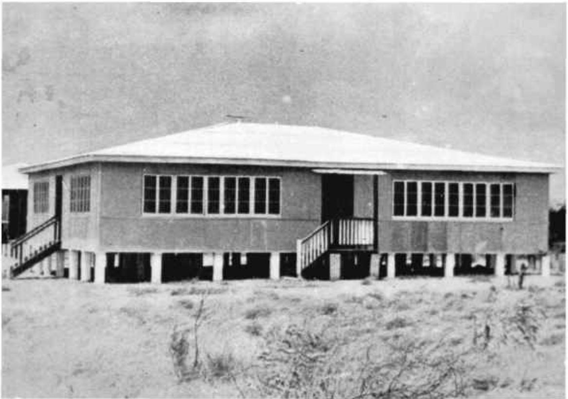
Islanders' Homes, Badu Island, under construction.
