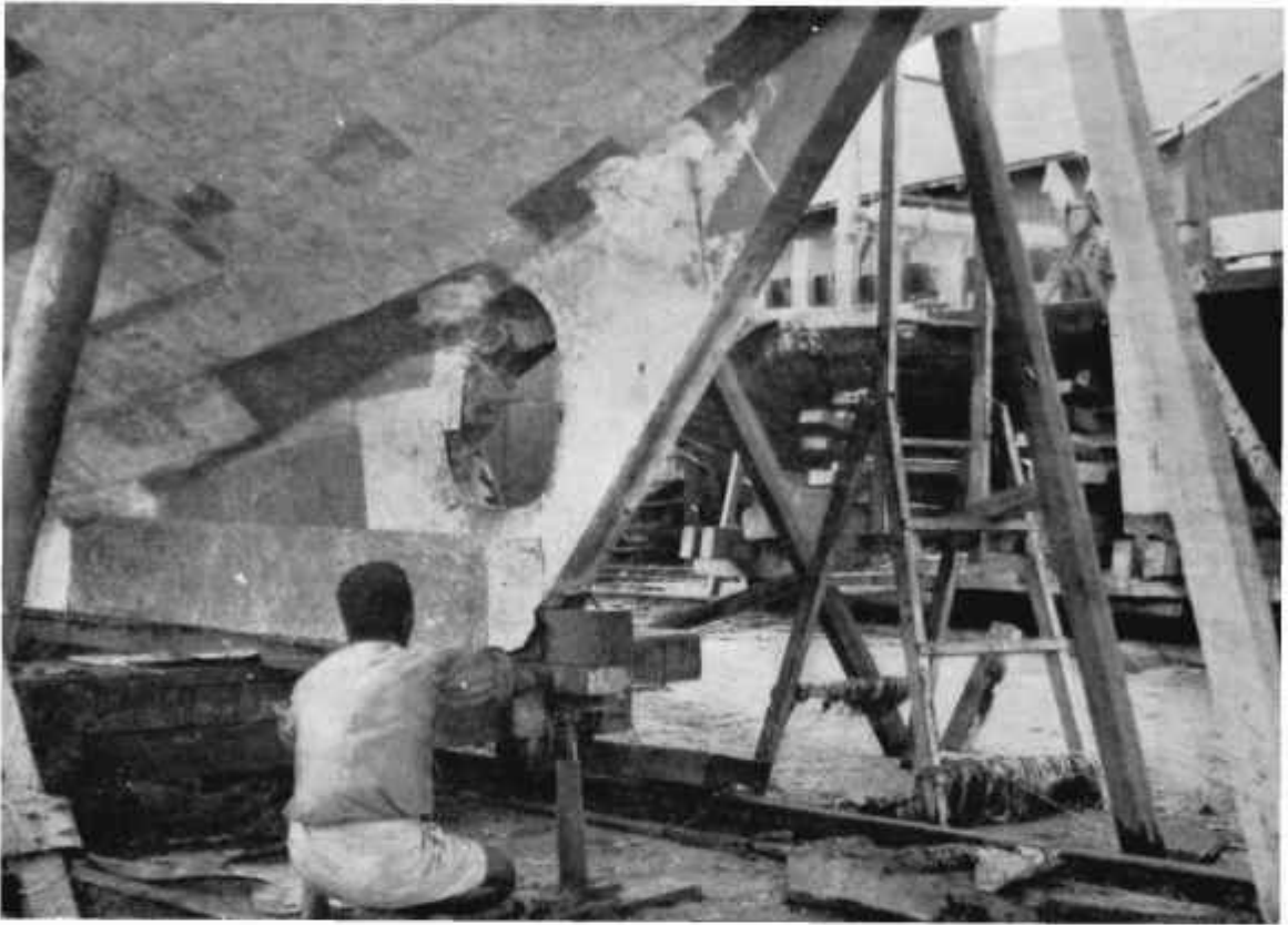
Recoppering Lugger I.I.B. Slipway.
