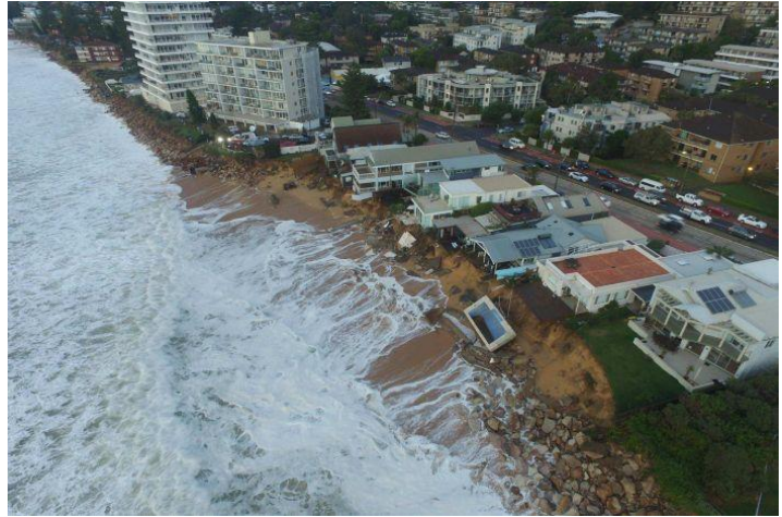
PHOTO: Waves have caused severe coastal erosion and damaged property. (Supplied: UNSW WRL)
