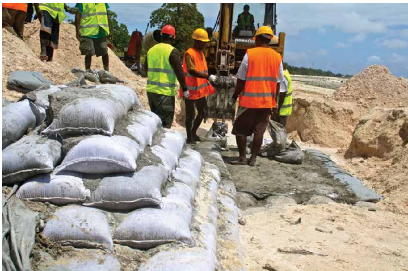
Building Seawalls. Tarawa, Kiribati.
