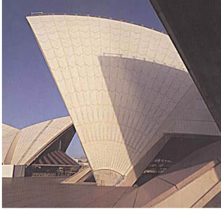
A view of the Concert Hall shell, with the shadow of the Opera Theatre shell across it and the restaurant shell in the background
