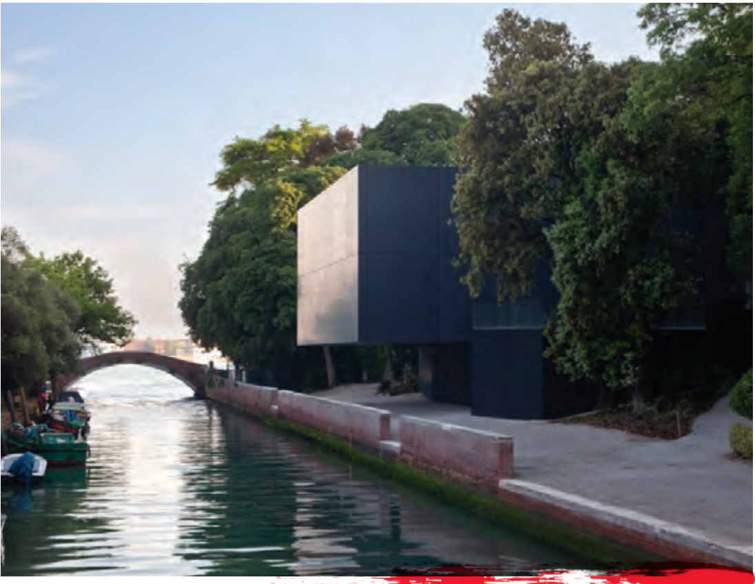
The new Australian Pavilion. Image credit: Alessandra Bello
