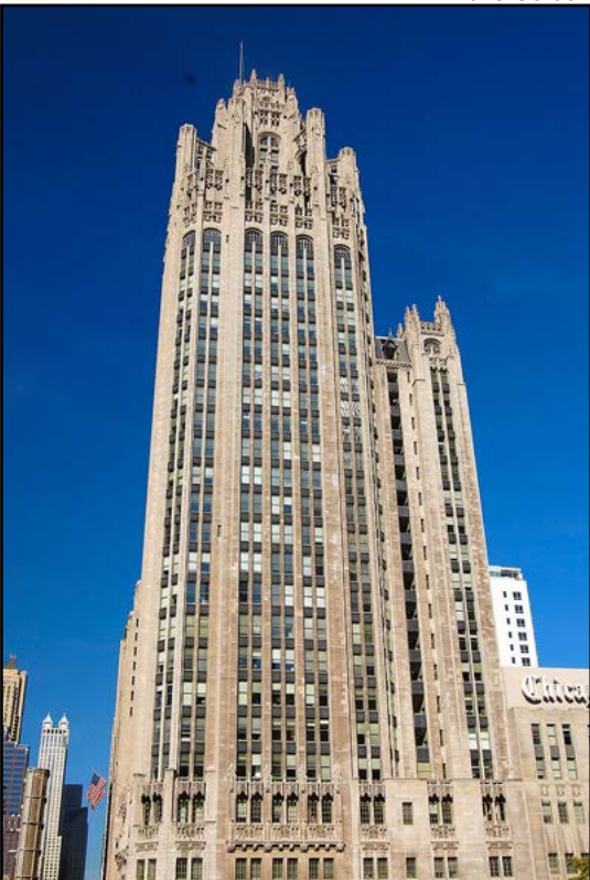
Figure 65 • Chicago Tribune Building (1922, Raymond Hood and John Mead Howells)
