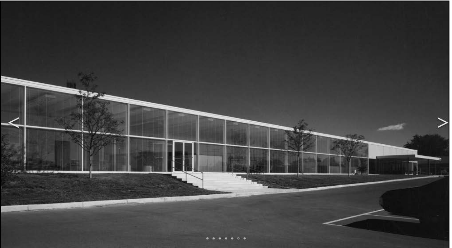
Figure 73 • Republic Newspaper Plant and Office, Columbus, Indiana (1971, SOM)
