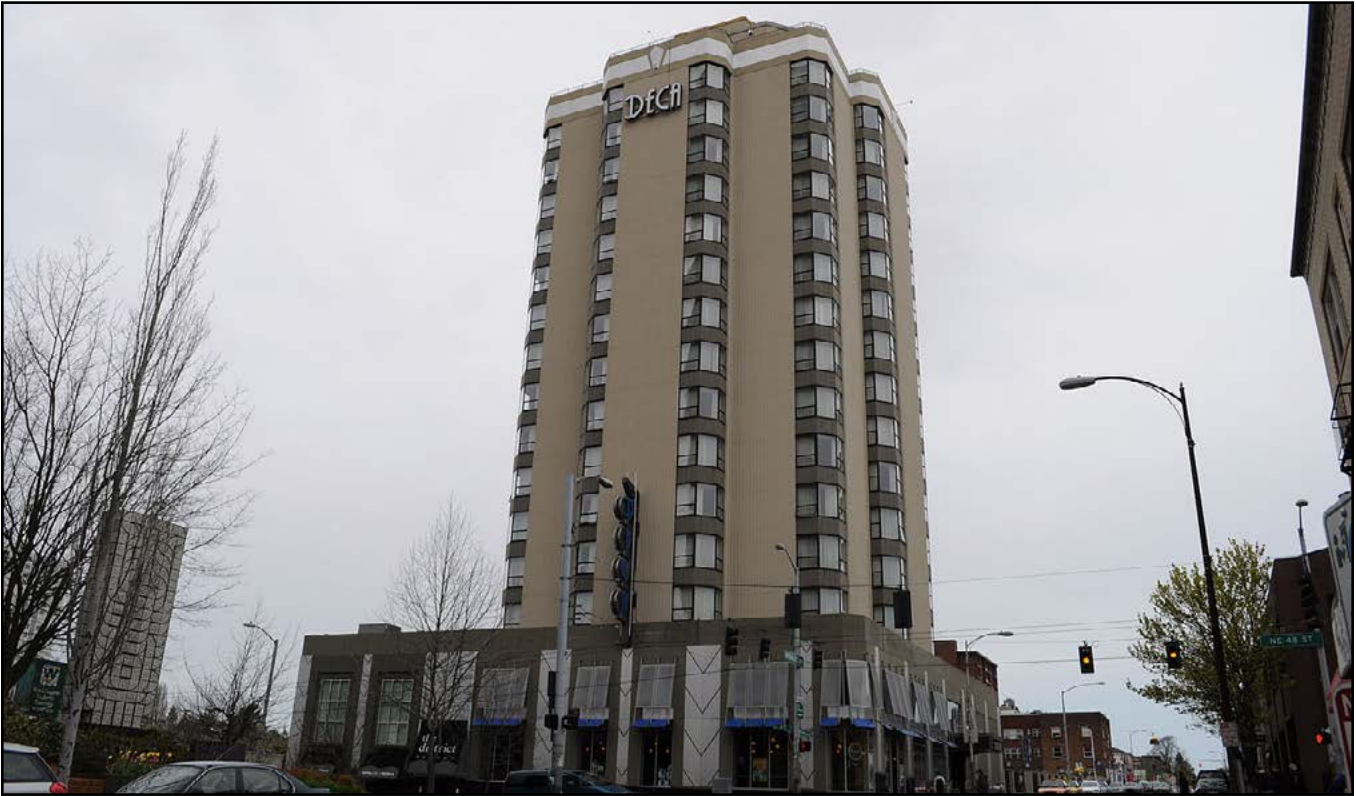
Figure 79 • Edmund Meany Building, Seattle (1926, Robert C. Reamer, Teufel & Carlson, contractors)
