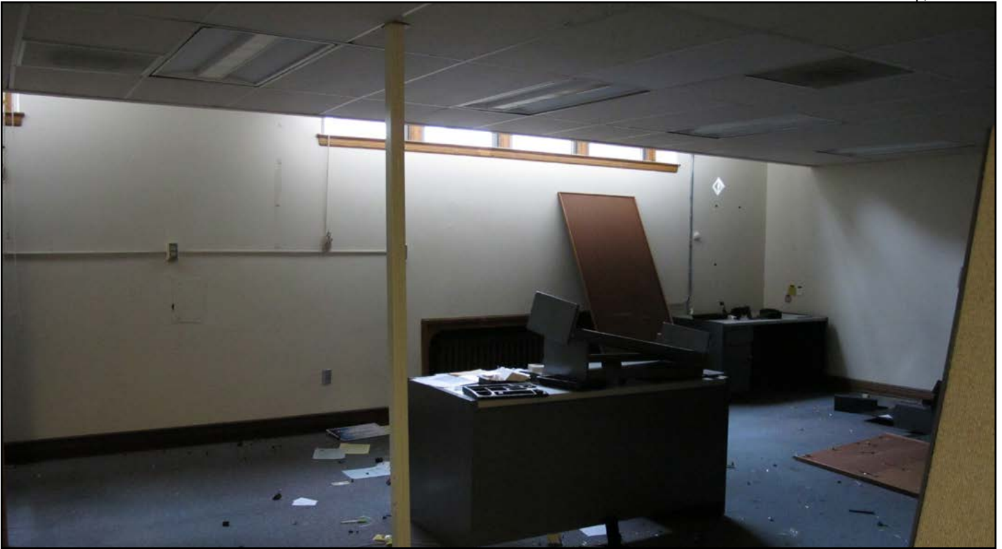
Figure 19 • Seattle Times Building Complex, 1947 Office Building Addition, interior at lower floor
