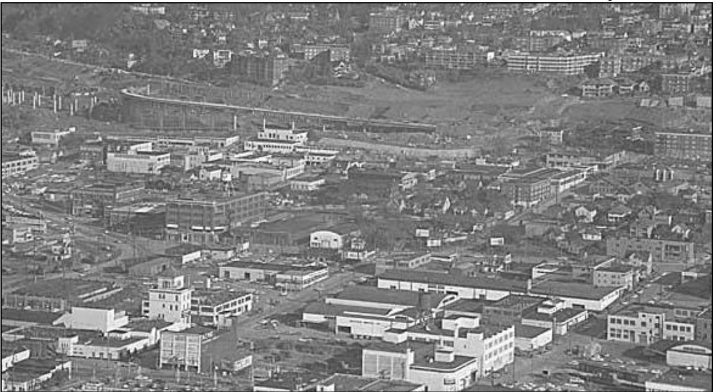
Figure 38 • South Lake Union viewing toward freeway construction from Space Needle, 1962
