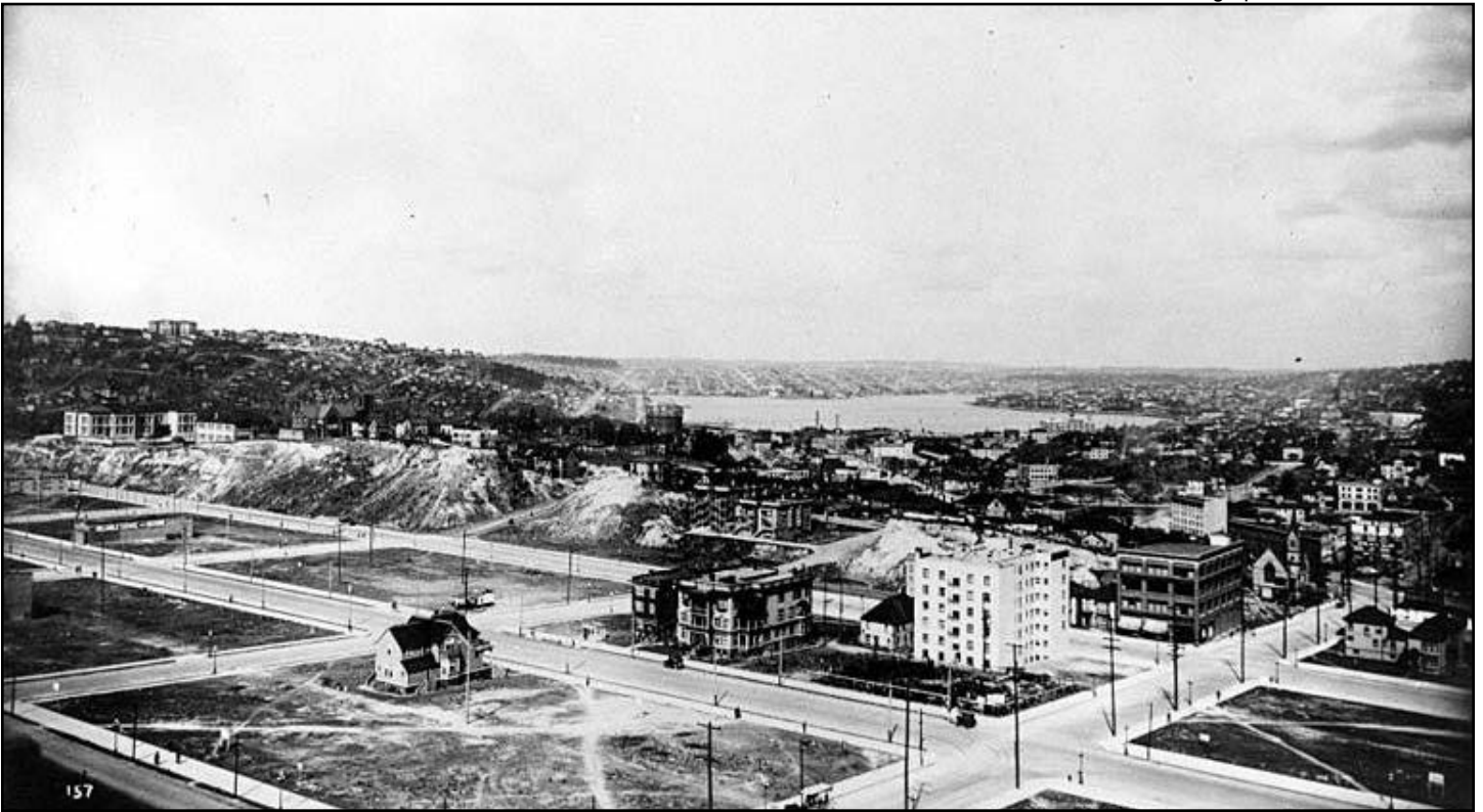
Figure 31 • Final Denny Re-grade viewing northeast, ca. 1930
