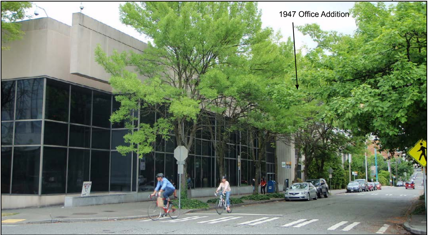
Figure 3 • View A - Viewing northeast from the corner of Boren Avenue N and John Street
