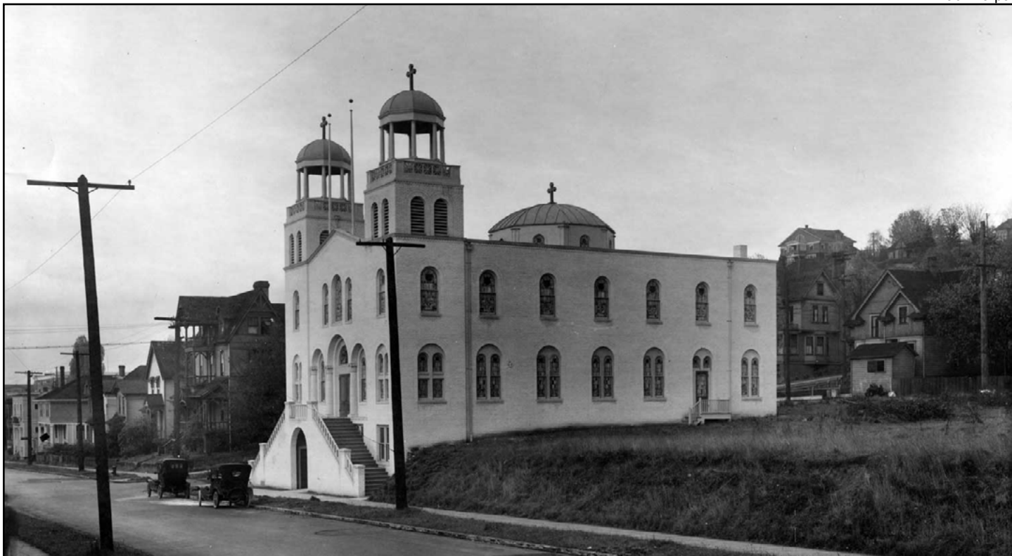
Figure 29 • St. Demetrios Greek Orthodox Church (1921, demolished)
