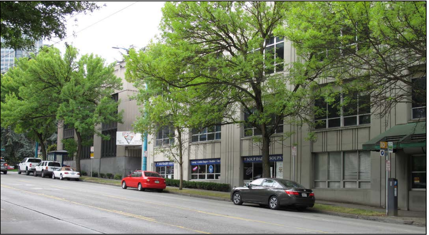
Figure 7 • View E - Viewing southeast from Fairview Avenue N
