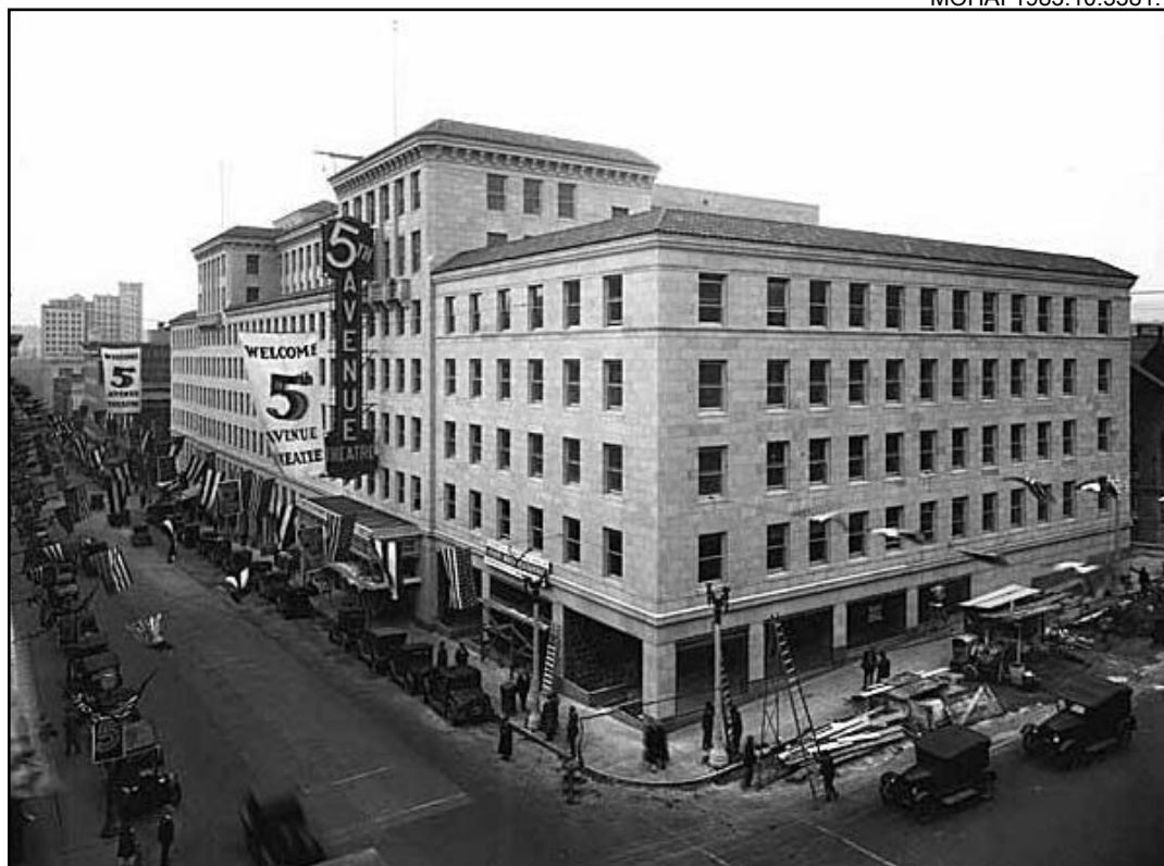
Figure 78 • Skinner Building, Seattle (1925-26, Robert C. Reamer, Teufel & Carlson, contractors)
