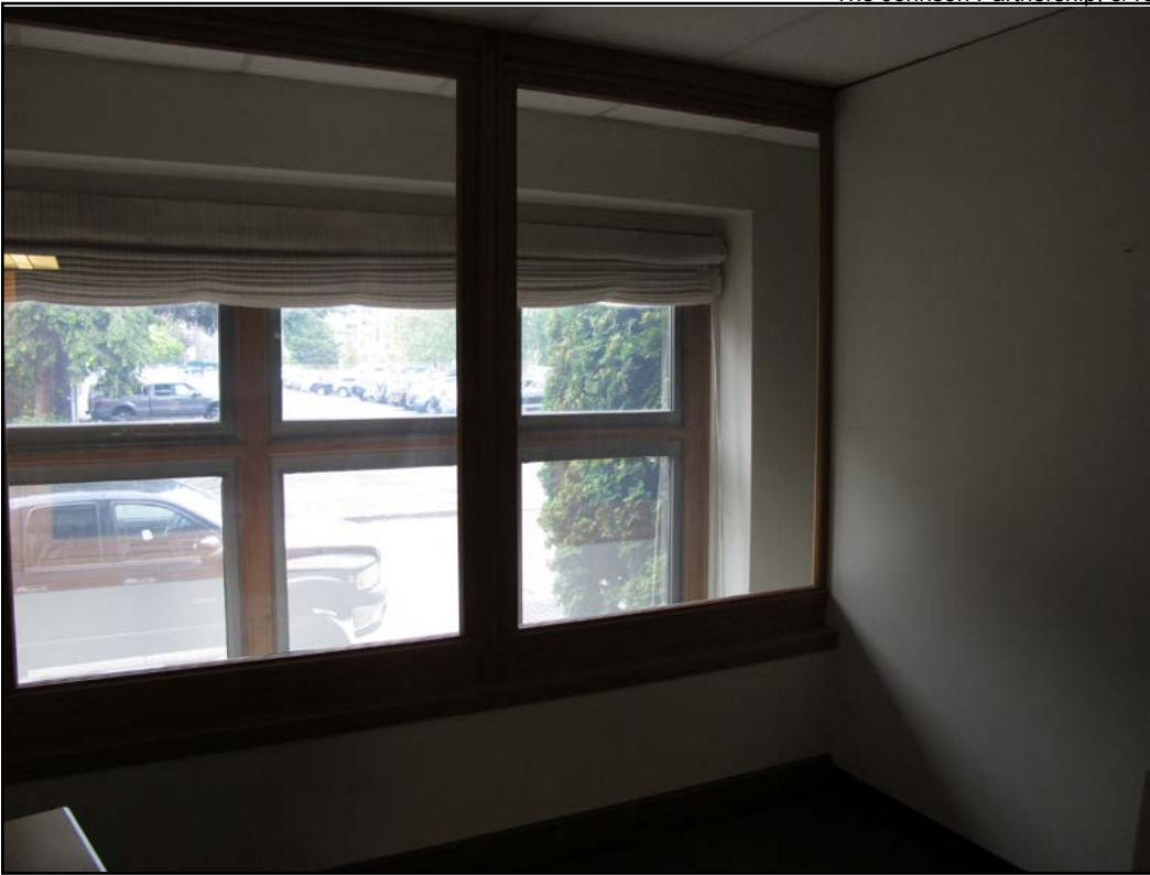
Figure 16 • Seattle Times Building Complex, 1947 Office Building Addition, interior at upper floor
