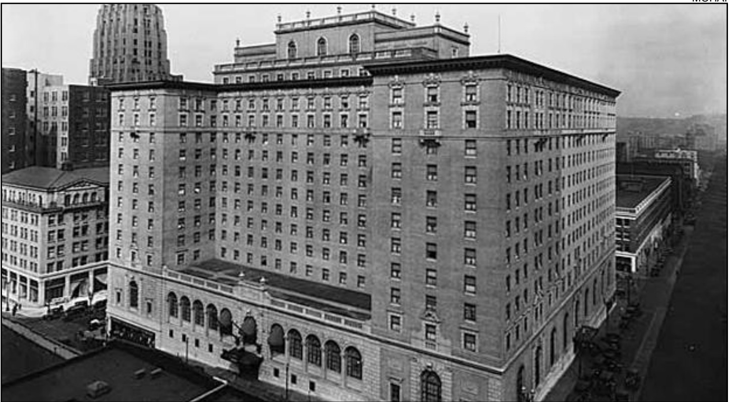
Figure 80 • Olympic Hotel (1924, George P. Post & Sons, Teufel & Carlson, contractors)
