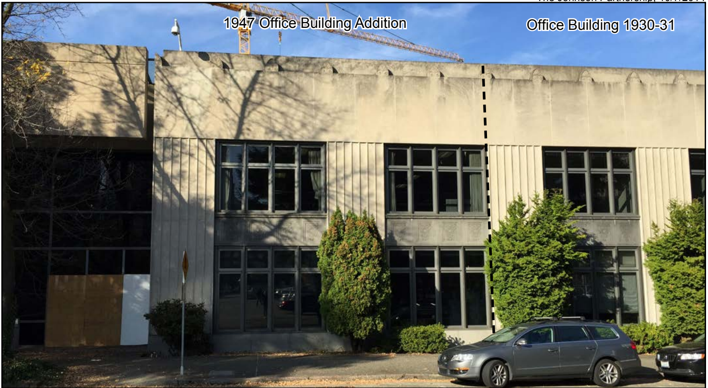
Figure 11 • Seattle Times Building Complex, 1947 Office Building Addition
