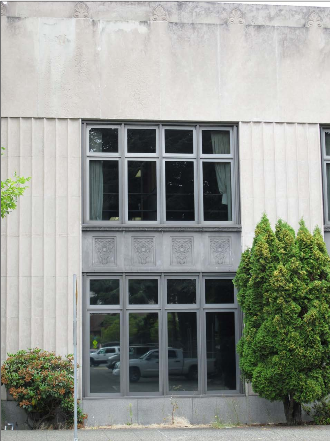
Figure 12 • Seattle Times Building Complex, 1947 Office Building addition, detail
