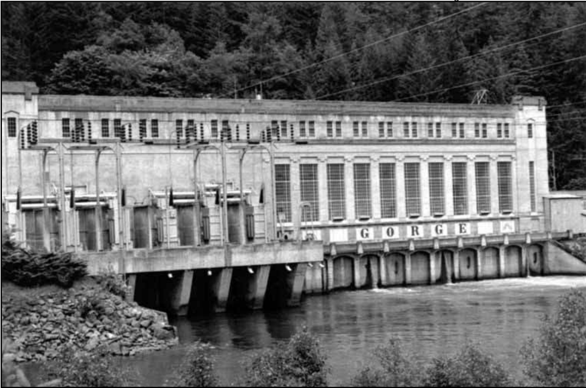
Figure 83 • Seattle City Light Gorge Powerhouse (1937, Teufel & Carlson, contractors, National Register District)
