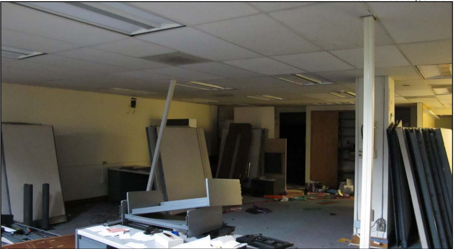
Figure 20 • Seattle Times Building Complex, 1947 Office Building Addition, interior at lower floor
