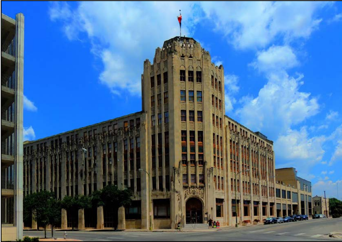
Figure 67 • San Antonio News Express Building (1929, Herbert S. Green)
