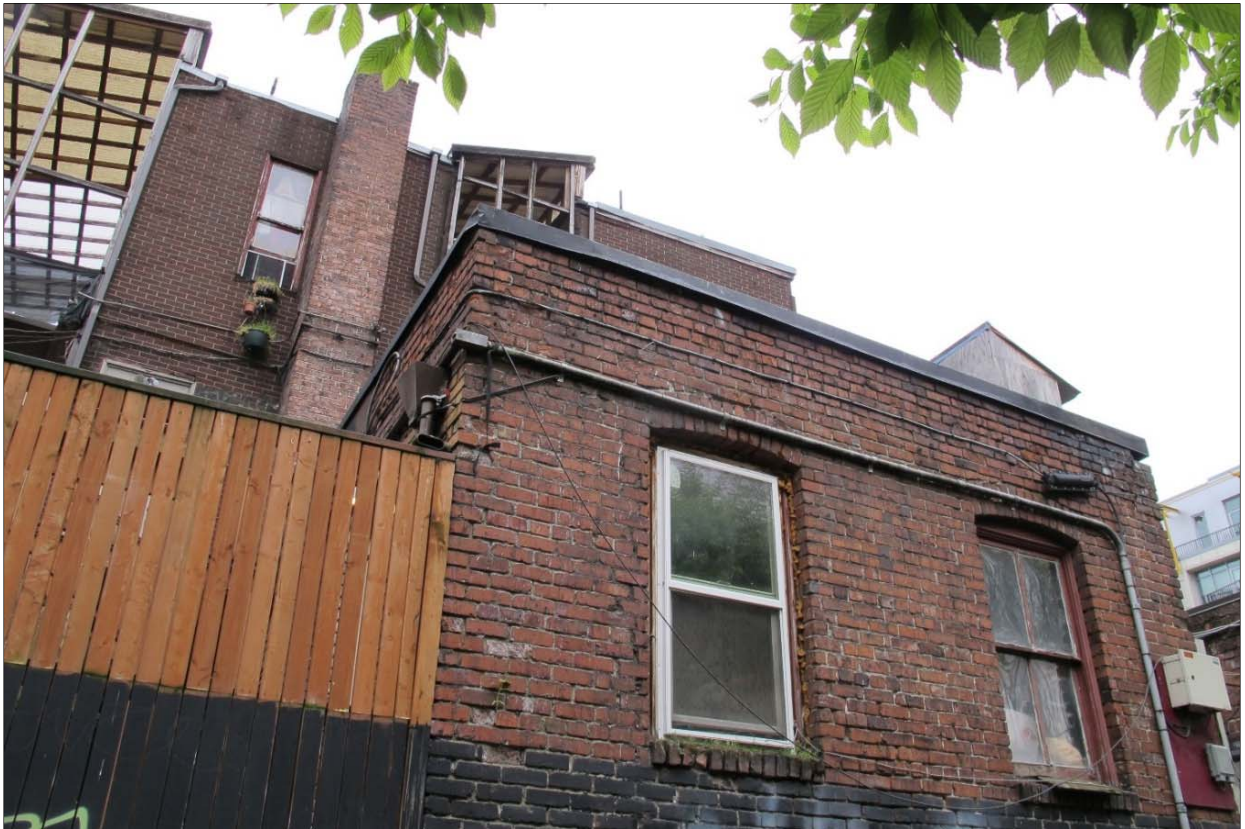
Fig. 70 – East elevation, partial view.
