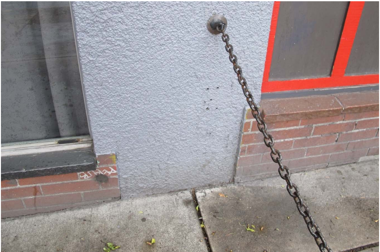
Fig. 58 – West elevation of storefronts, detail.
