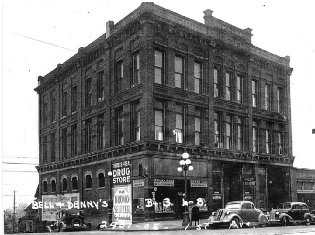
Fig. 6 – Hull Building, built 1889, at the northwest corner of First and Battery. (1937 tax assessor photo)
