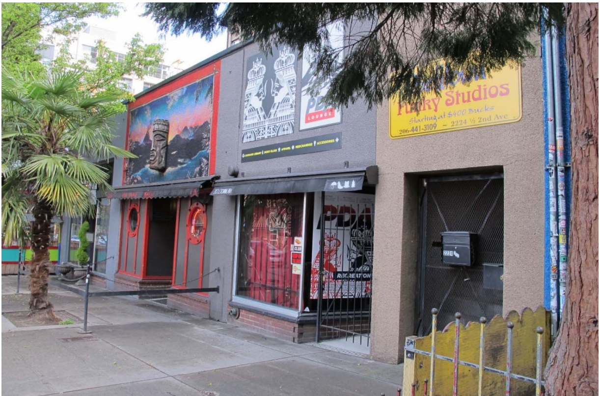
Fig. 60 – West elevation of storefronts.
