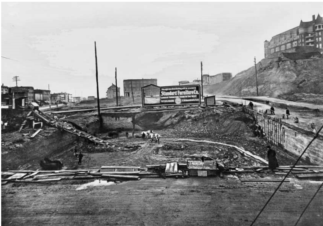
Fig. 17 – Circa 1906 view of regraded First and Second Avenues at Pine Street, looking north. (www.pauldorpat.com; UWSC JEW0852 sim.)
