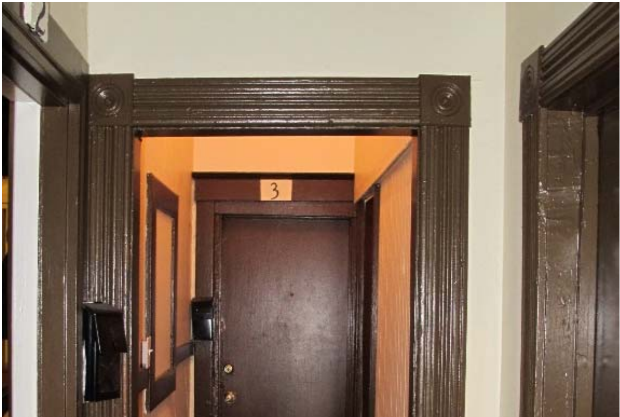
Fig. 78 – Interior, typical door trim in corridor.
