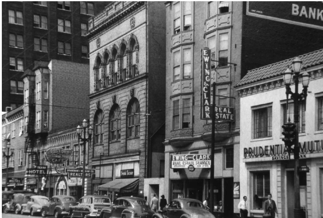
Fig. 34 – Charles L. Haynes: Pacific Telephone building alteration (1908).
