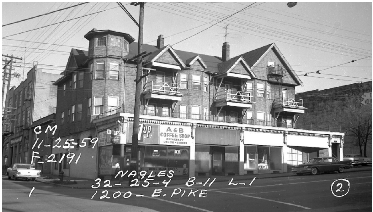
Fig. 32 – Rowhouse-like building at 1200 E. Pike (demolished), with commercial floor at sidewalk level inserted following the widening and regrade of Pike Street c. 1911. (1959 tax assessor photo)
