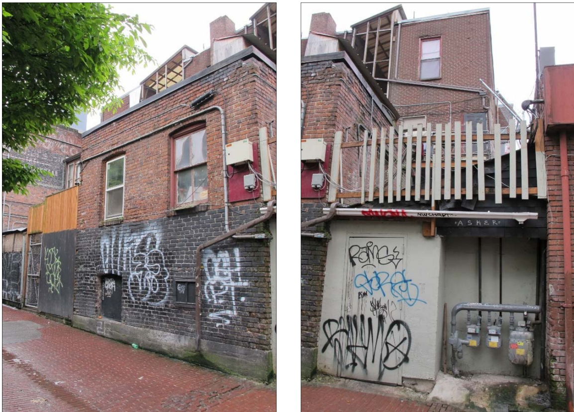
Fig. 68 – East elevation, partial view (middle and northernmost thirds)
