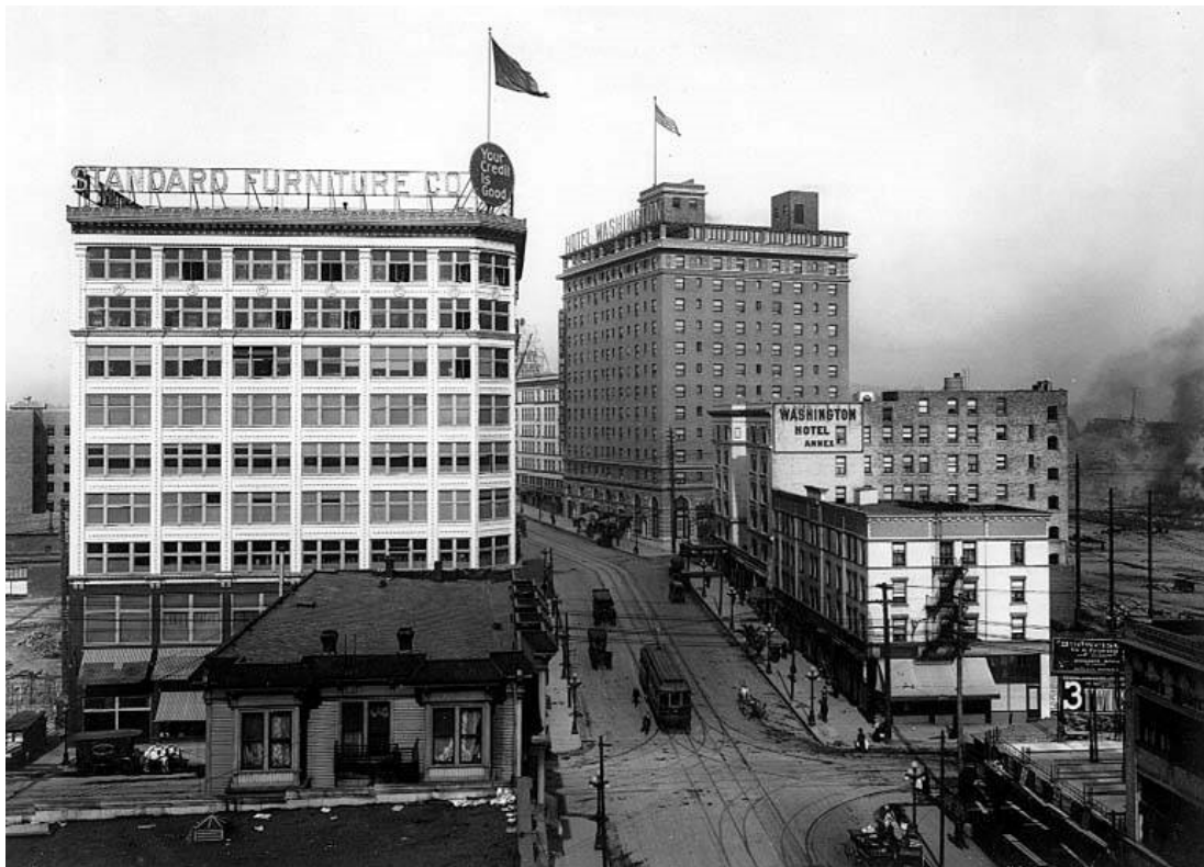
Fig. 21 – Circa 1909 view north along regraded Second Avenue, at Pike and Pine. (UWSC CUR683)
