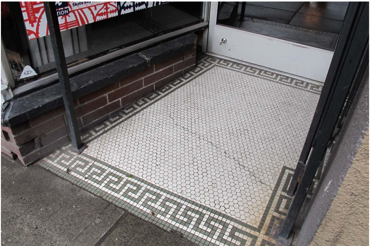
Fig. 59 – West elevation of storefronts, detail.
