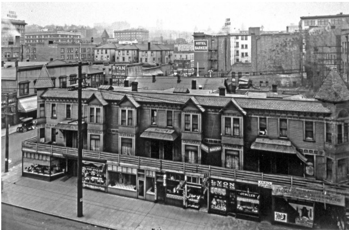
Fig. 31 – Rowhouses at the southwest corner of Pine and Sixth, with commercial floor at sidewalk level inserted following the regrade of Pine Street c.1905. (www.pauldorpat.com)
