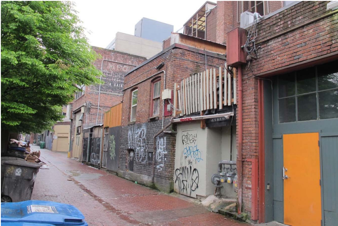
Fig. 65 – East elevation, partial view.
