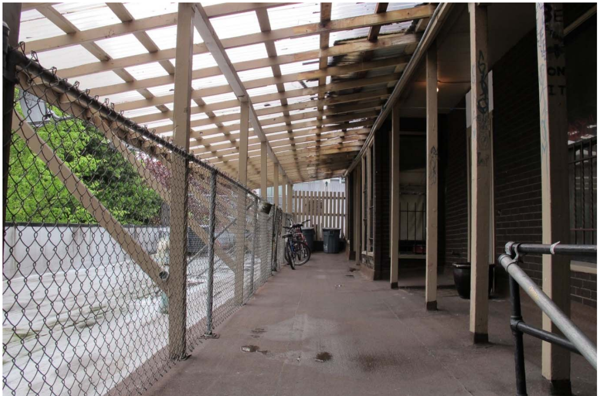
Fig. 72 – Roof deck at front (west side) of second floor residential level.
