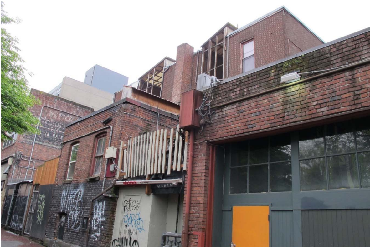
Fig. 66 – East elevation, partial view.
