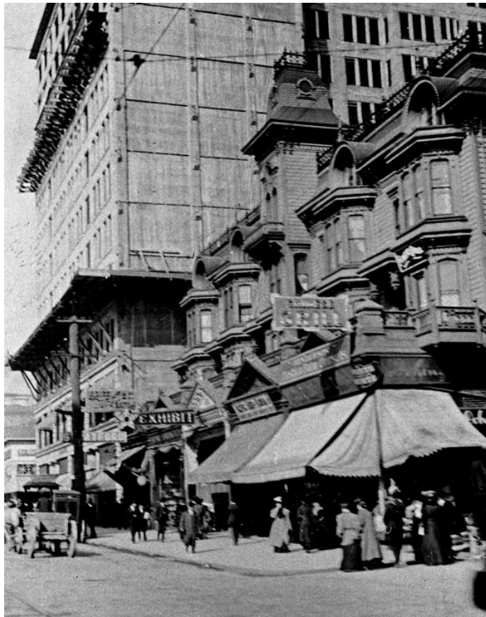
Fig. 23 – Stetson & Post rowhouses, c. 1905, showing commercial floor added at sidewalk level. (Michael Maslan, www.pauldorpat.com )
