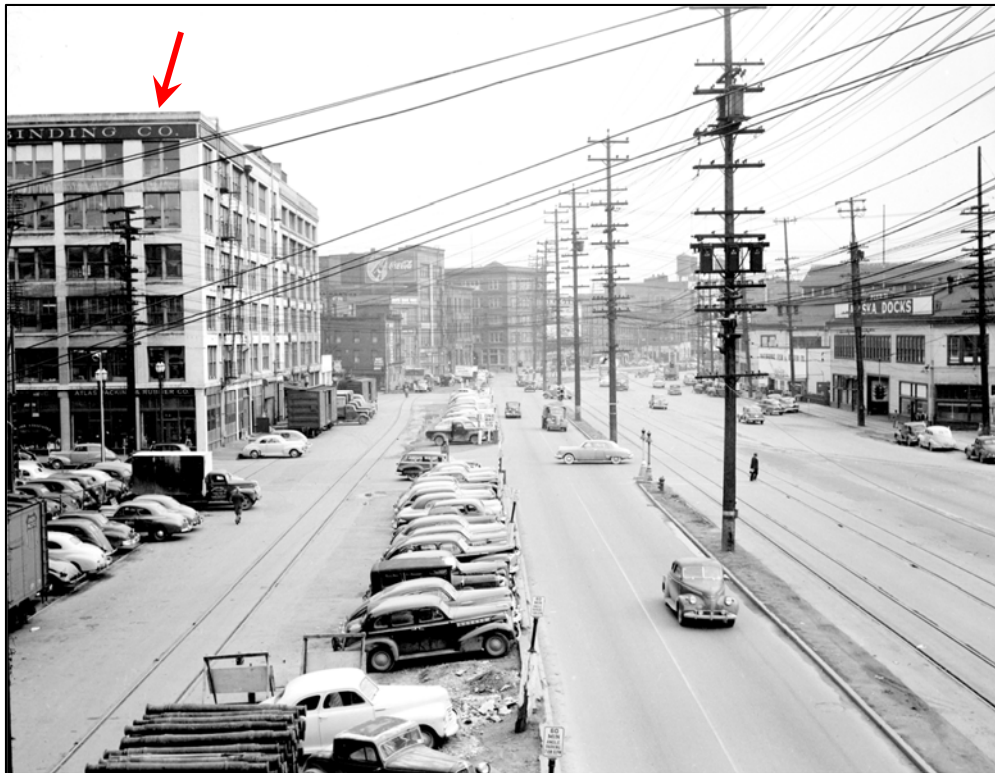
Fig. 24 – 1948 view, subject building at left. (SMA 42993)
