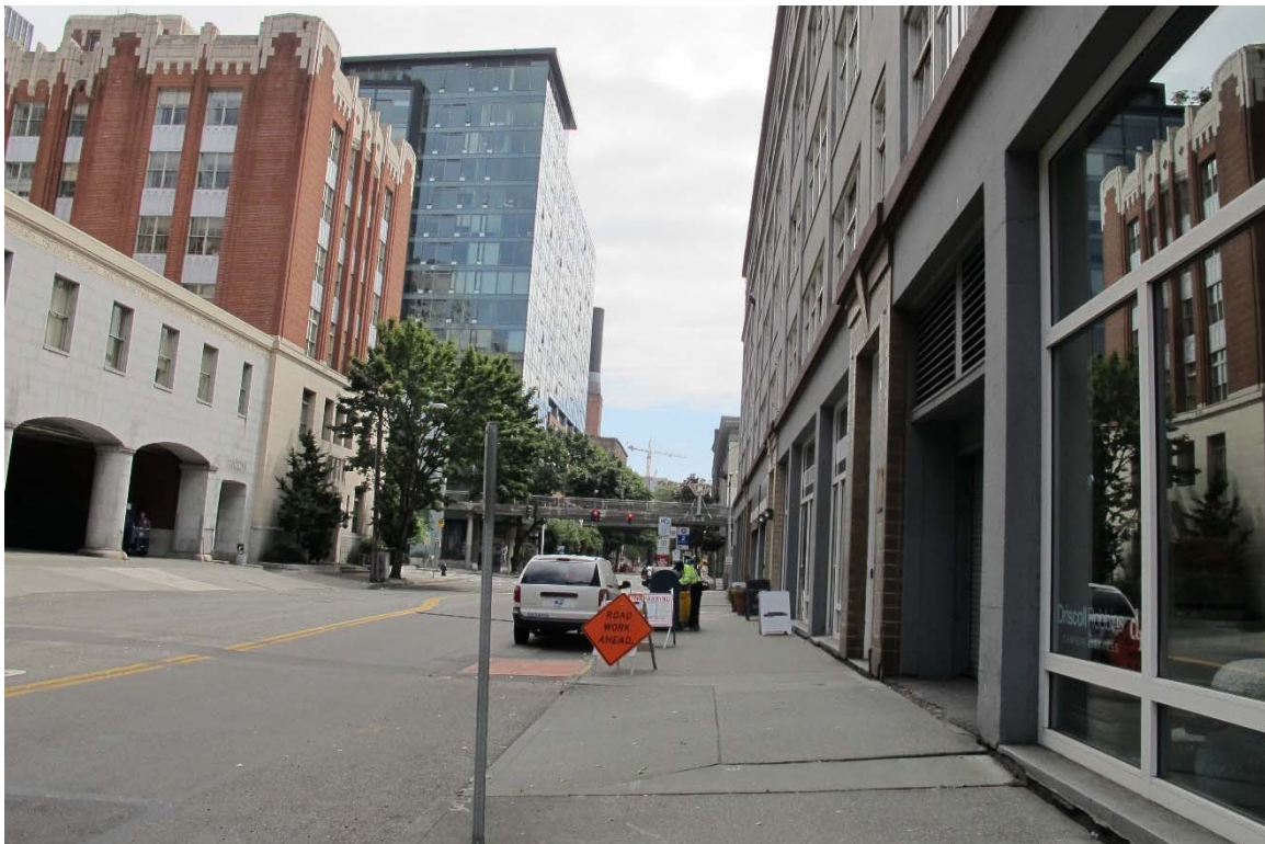
Fig. 63 – Detail, east elevation at sidewalk. Note modern storefronts and garage entry with transom vent.
