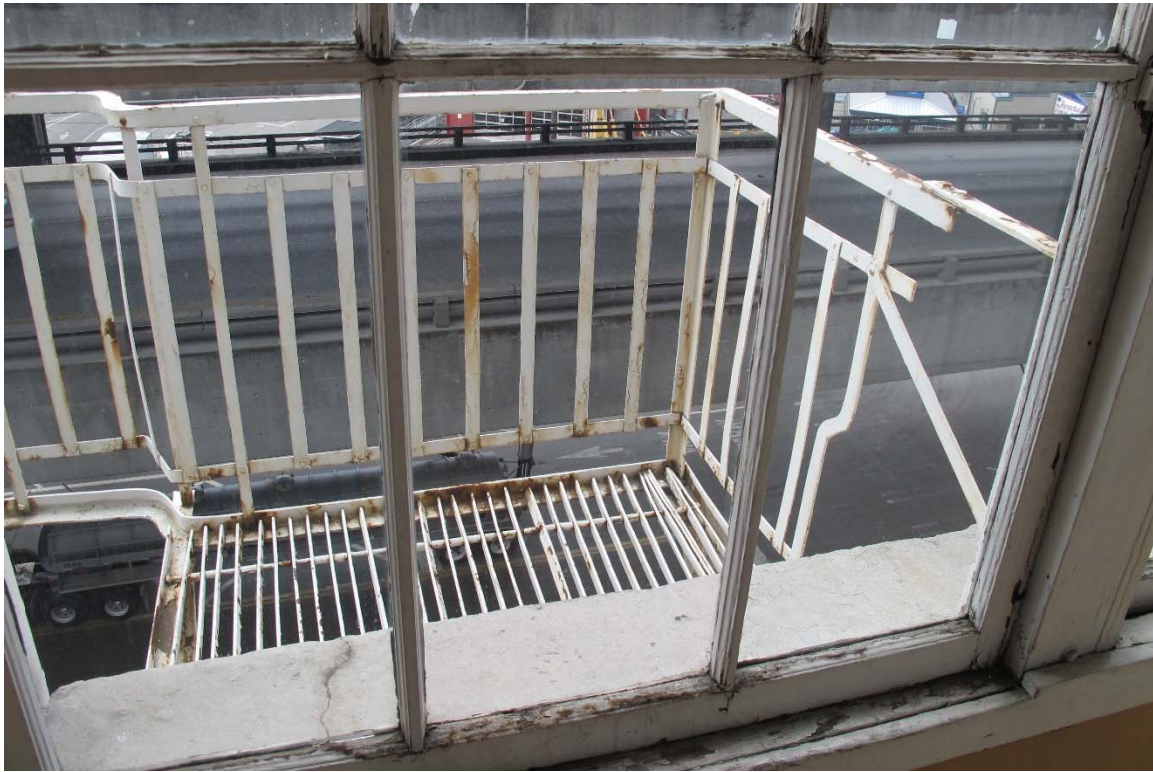
Fig. 70 – Interior, detail showing window and steel balconies on west elevation.
