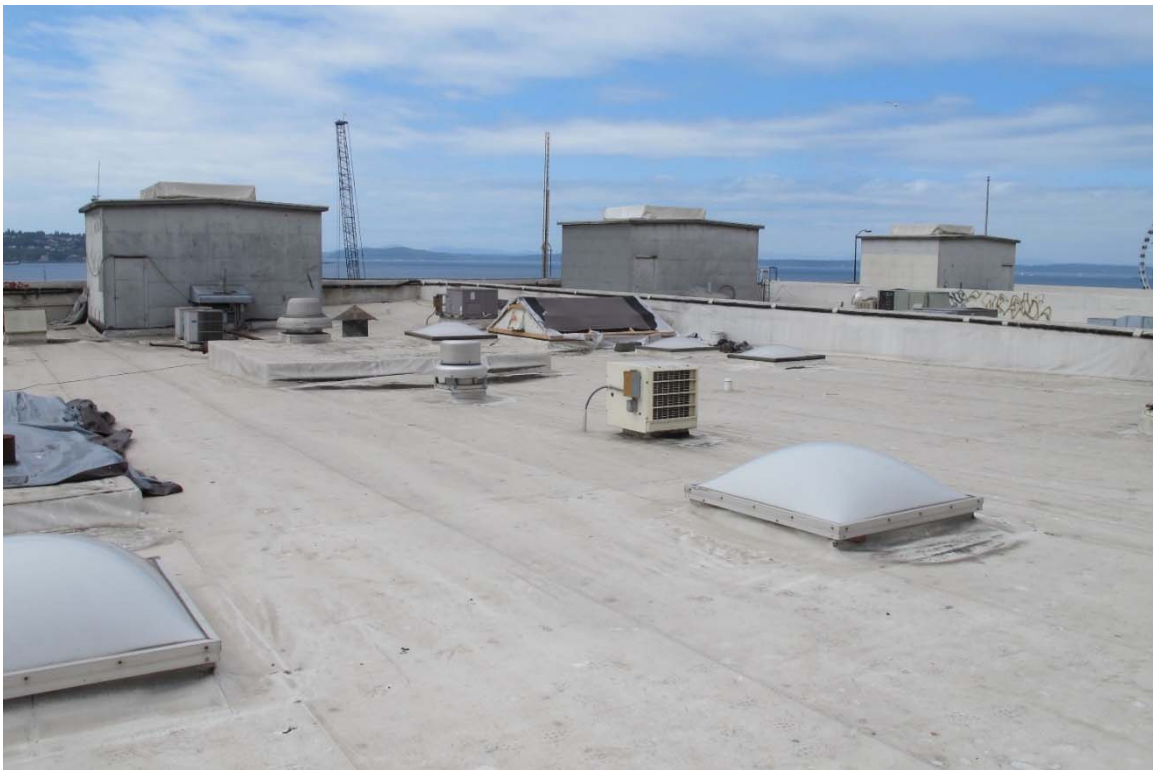
Fig. 71 – Roof, showing freight elevator penthouses along west side of building.
