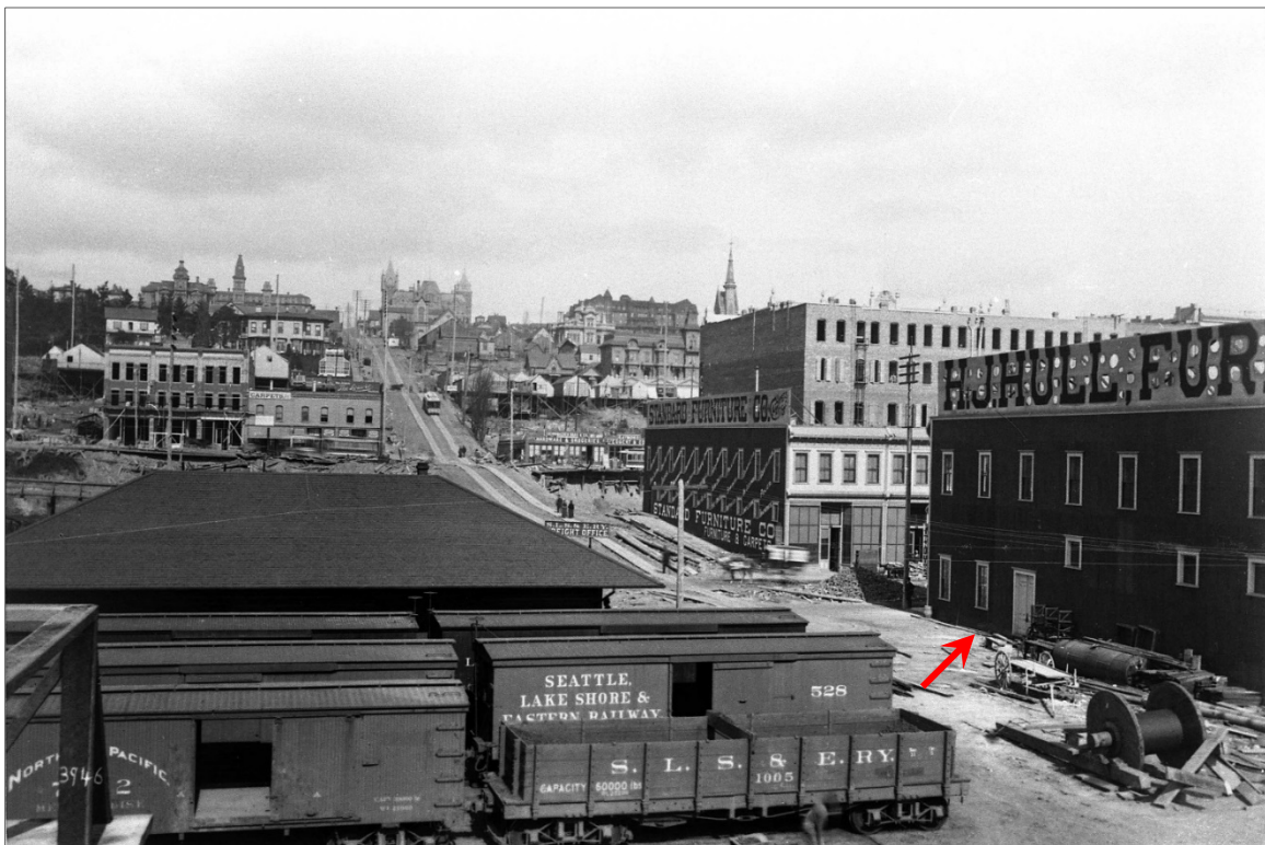
Fig. 6 – 1890 view of Madison Street, during rebuilding following the Great Fire. Subject site indicated by arrow, here occupied by the structure which existed before the subject building. (UWSC SEA0657)
