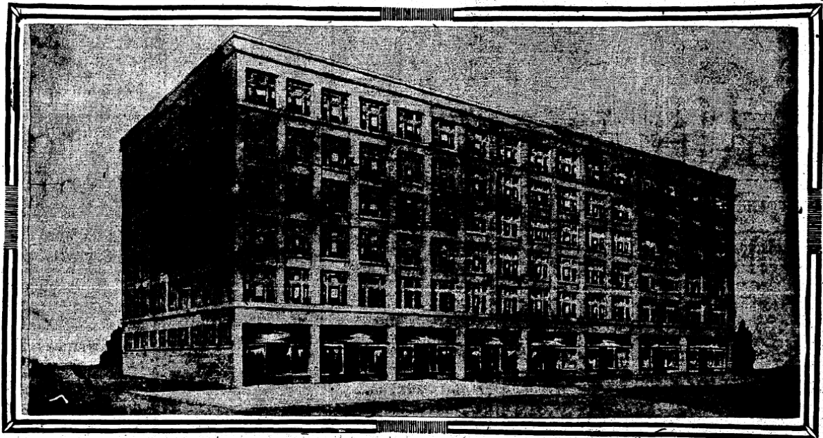
Fig. 43 – An early proposal for the subject building, which would have been six stories, and having no frontage on Marion and Madison Streets. No architect was listed. (Seattle Times, August 22, 1909).
