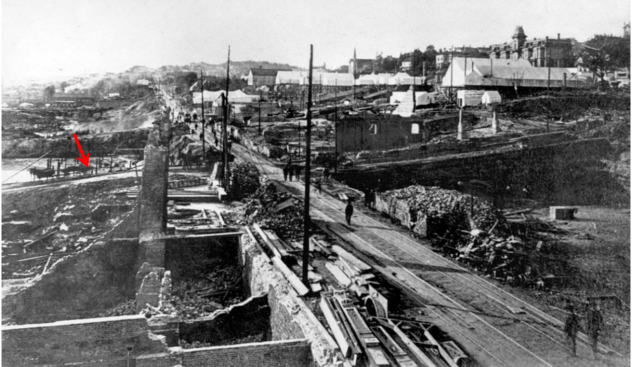
Fig. 5 – 1889 view after the Great Fire. Subject site, between Madison and Marion Streets, indicated by arrow. (www.pauldorpat.com)
