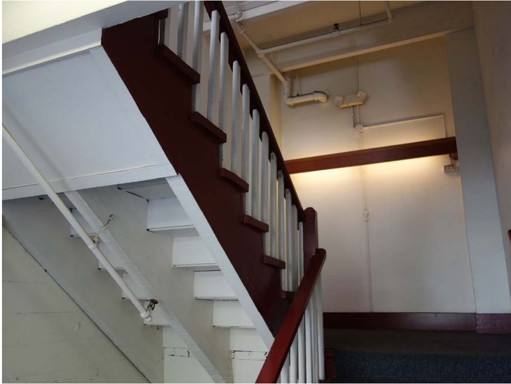
Fig. 68 – Interior, typical stair accessed from Western Avenue. (Bassetti Architects photo)
