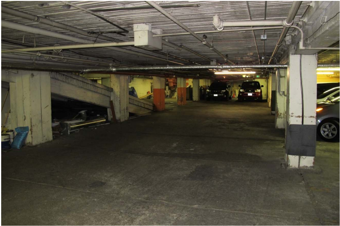
Fig. 80 – Interior, basement parking garage.
