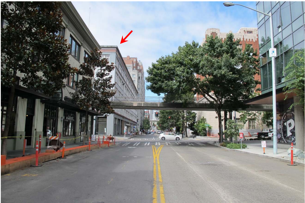
Fig. 47 – Context: View northward on Western Avenue; subject building indicated by arrow.
