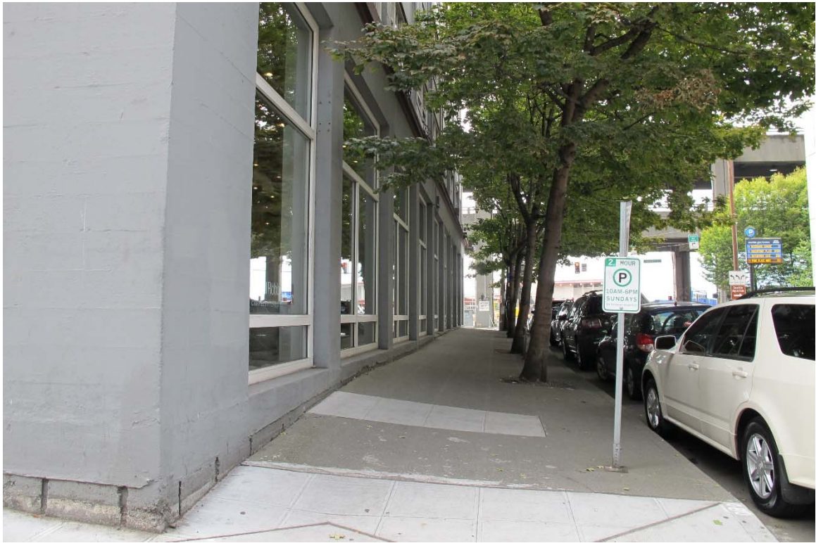
Fig. 64 – Detail, north elevation at sidewalk.
