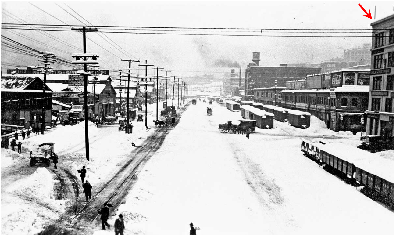
Fig. 20 – 1916 view showing docks. Subject building at right. (www.pauldorpat.com)
