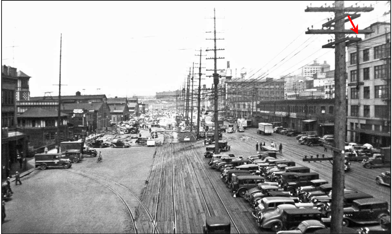
Fig. 23 – 1936 view of Alaskan Way/Railroad Avenue, subject building at right. (www.pauldorpat.com)
