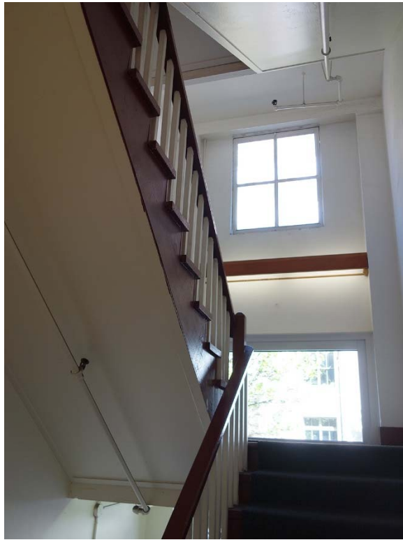
Fig. 69 – Interior, typical stair accessed from Western Avenue. (Bassetti Architects photo)
