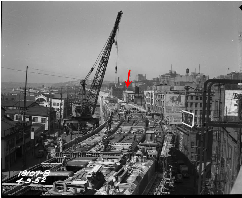
Fig. 25 – 1952 view of construction of Alaskan Way Viaduct. Subject building indicated by arrow. (SMA SMA43549)
