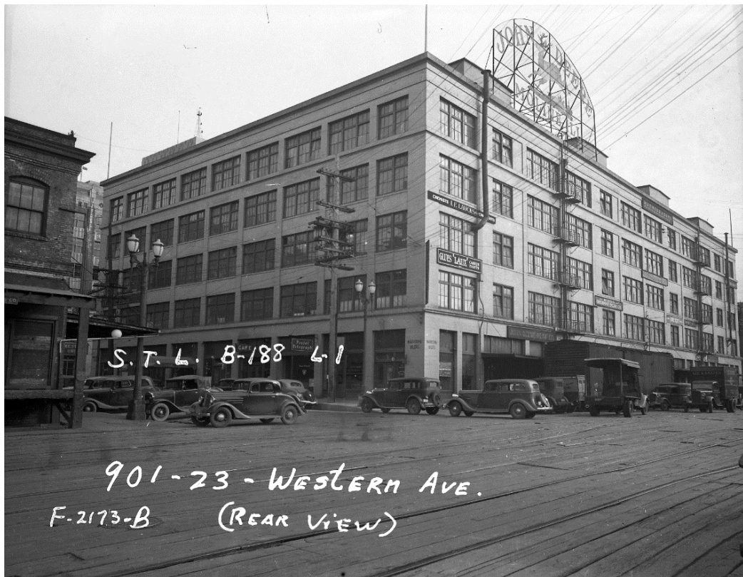
Fig. 45 – 1937 tax assessor photo showing the northwest corner of the building.
