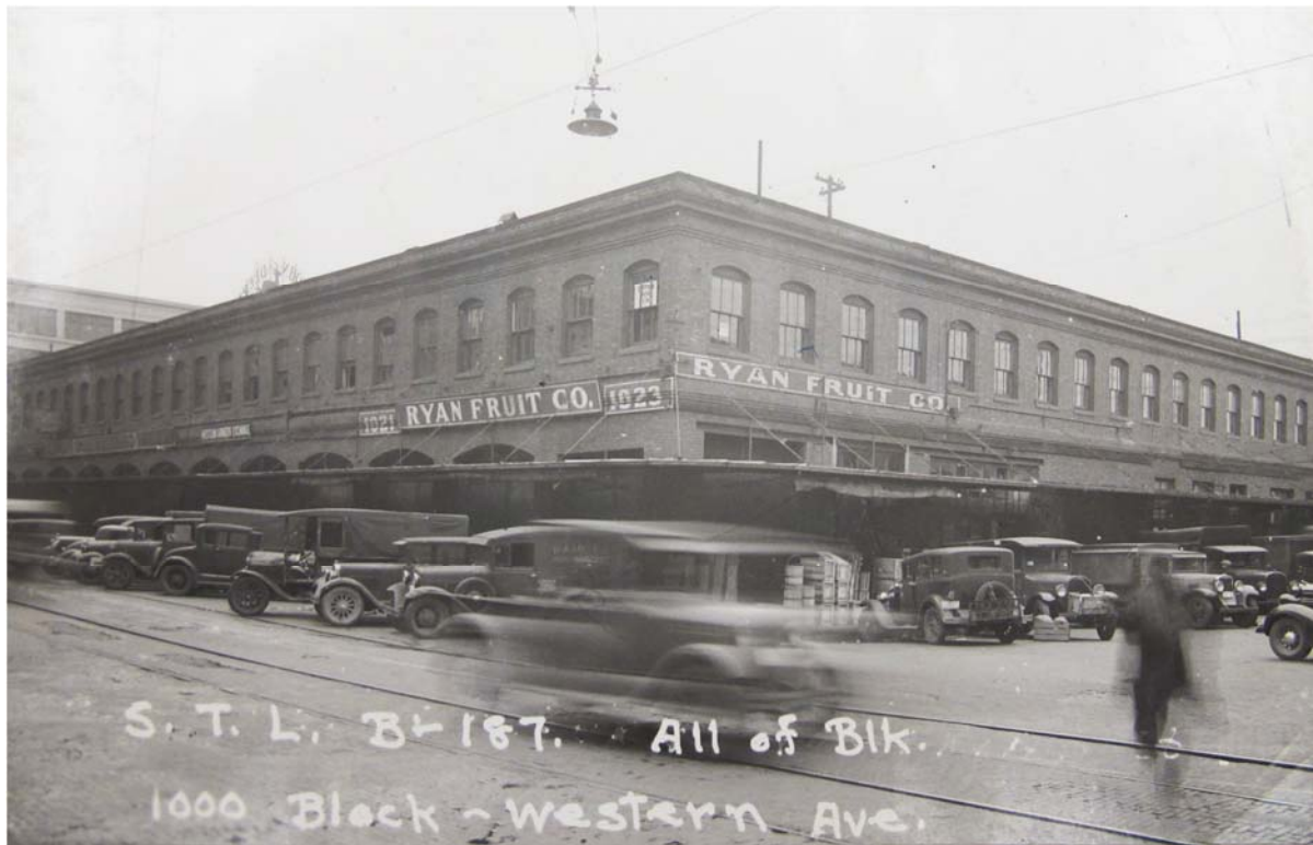
Fig. 30 – View of the warehouse building which was directly north of the subject building and occupied the entire block, in 1937 (no longer extant). This building was constructed by the Pacific Warehouse Company, the same developer of the subject site, in 1908-09. (Tax assessor photo)
