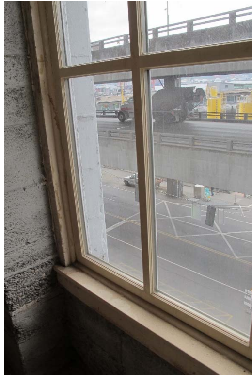
Fig. 78 – Interior, typical shell of office space, detail of demising wall (left) and replacement wood sash window (right).
