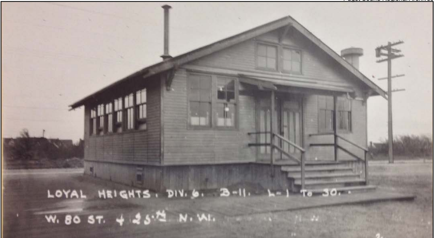
Figure 66. Loyal Heights School, portable classroom, ca. 1937
