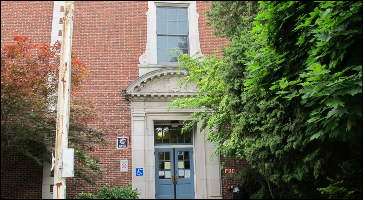
Figure 17. Loyal Heights Elementary School, northern façade, detail of eastern entry door
