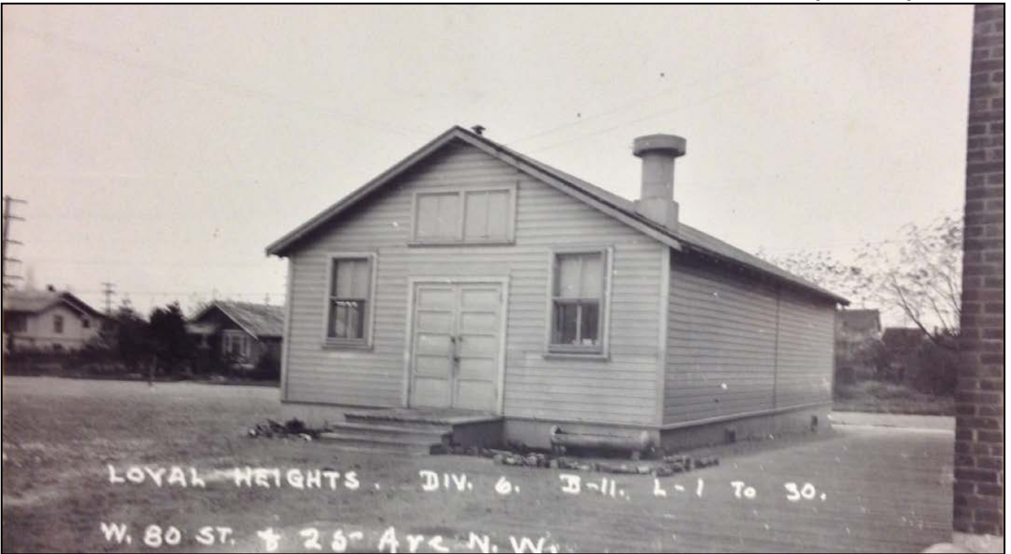
Figure 65. Loyal Heights School, portable classroom, ca. 1937
