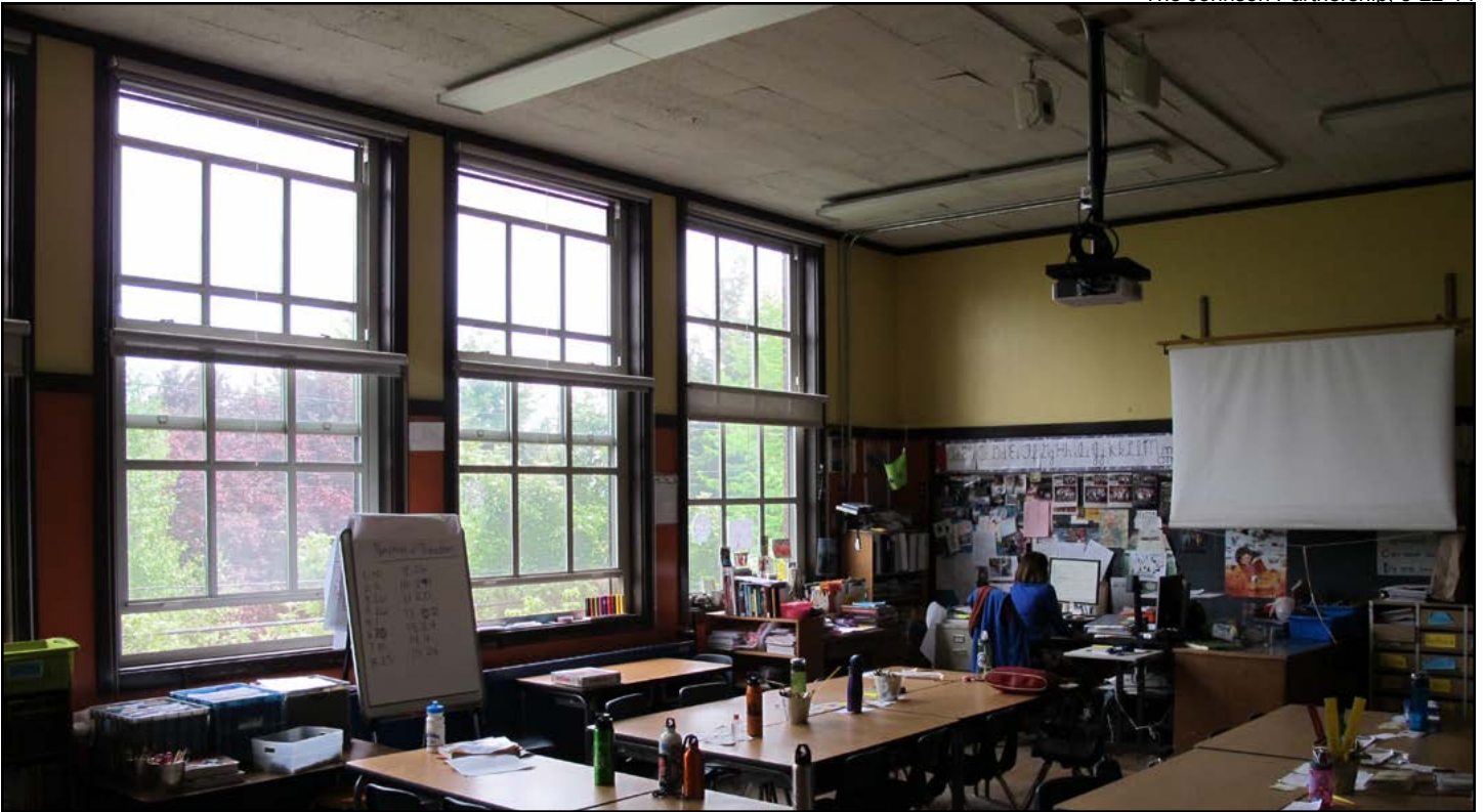
Figure 43. Loyal Heights Elementary School, typical second floor classroom
