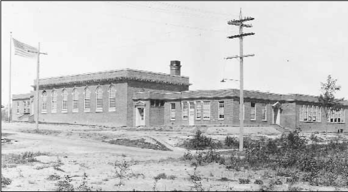
Figure 79. Highland Park School, 1012 SW Trenton Street (1921, Floyd A. Naramore, demolished 1998)
