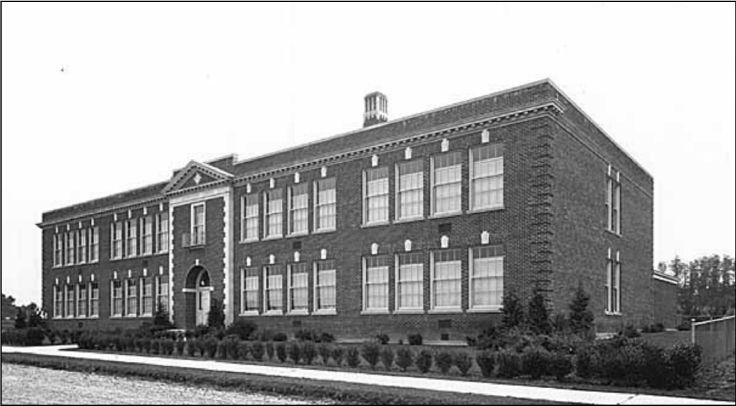
Figure 87. Laurelhurst School, 4530 46th Avenue NE (1928, Floyd A. Naramore, altered)
