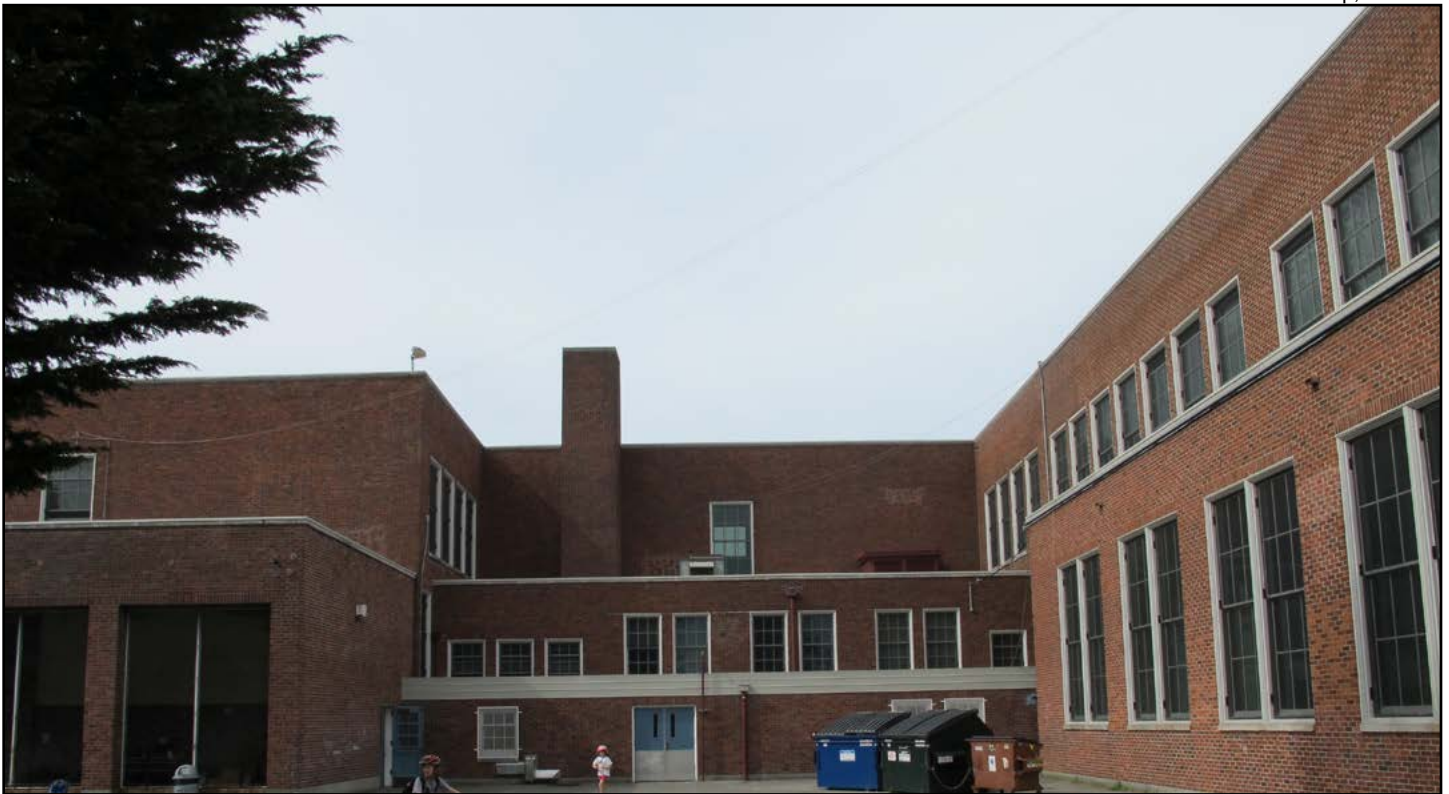
Figure 24. Loyal Heights Elementary School, southern façade, central portion
