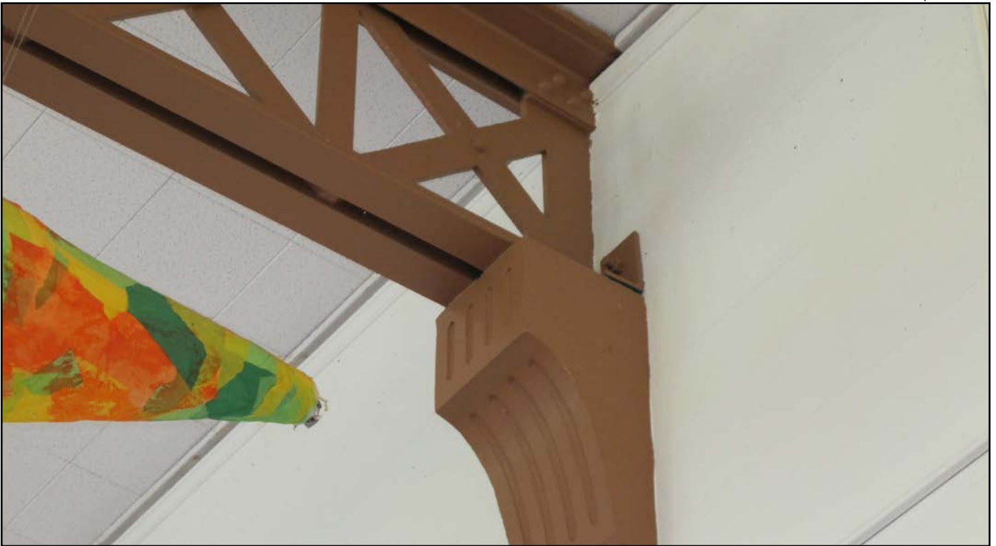
Figure 35. Loyal Heights Elementary School, detail at steel truss in auditorium/lunchroom
