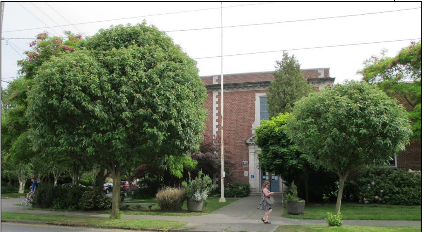
Figure 16. Loyal Heights Elementary School, northern façade, eastern entry door
