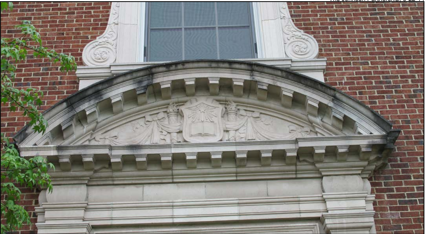
Figure 12. Loyal Heights Elementary School, northern façade, detail at western entry
