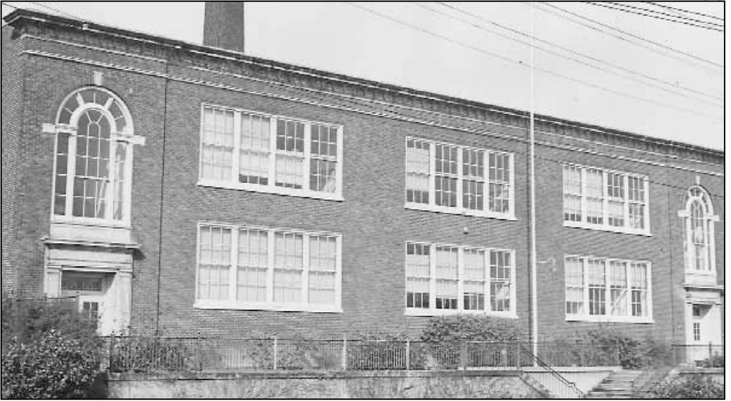
Figure 84. Montlake School, 2409 22nd Avenue E (1924, Floyd A. Naramore, Seattle Landmark)
