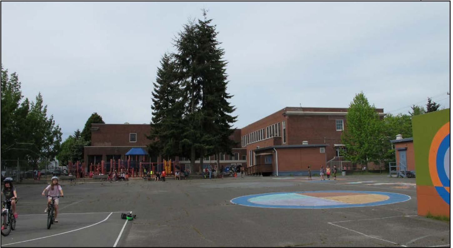
Figure 27. Loyal Heights Elementary School, southern façade, viewing across play area
