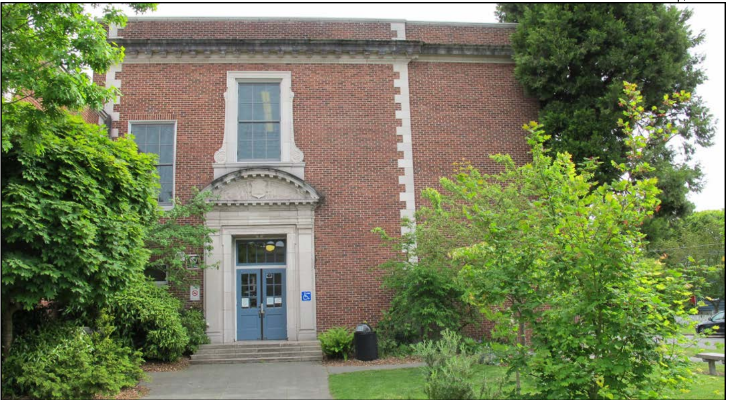
Figure 14. Loyal Heights Elementary School, northern façade, western entry door
