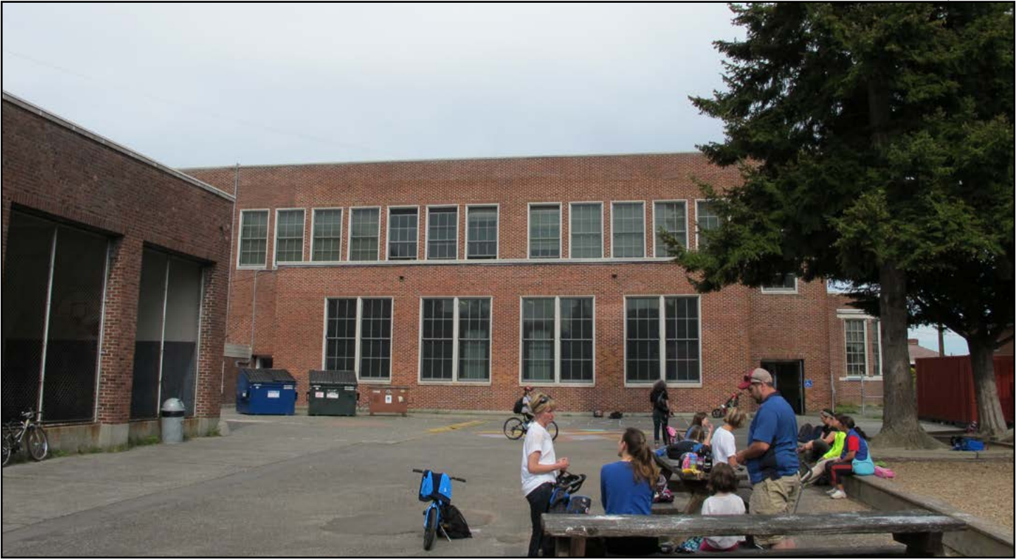
Figure 23. Loyal Heights Elementary School, western façade of eastern wing
