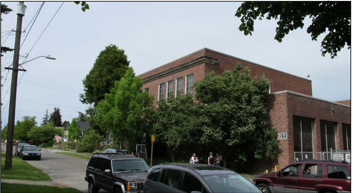
Figure 28. Loyal Heights Elementary School, western façade, viewing northeast
