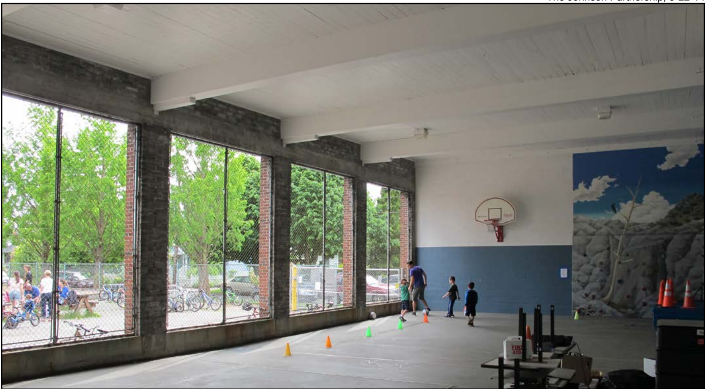
Figure 46. Loyal Heights Elementary School, covered play-courts
