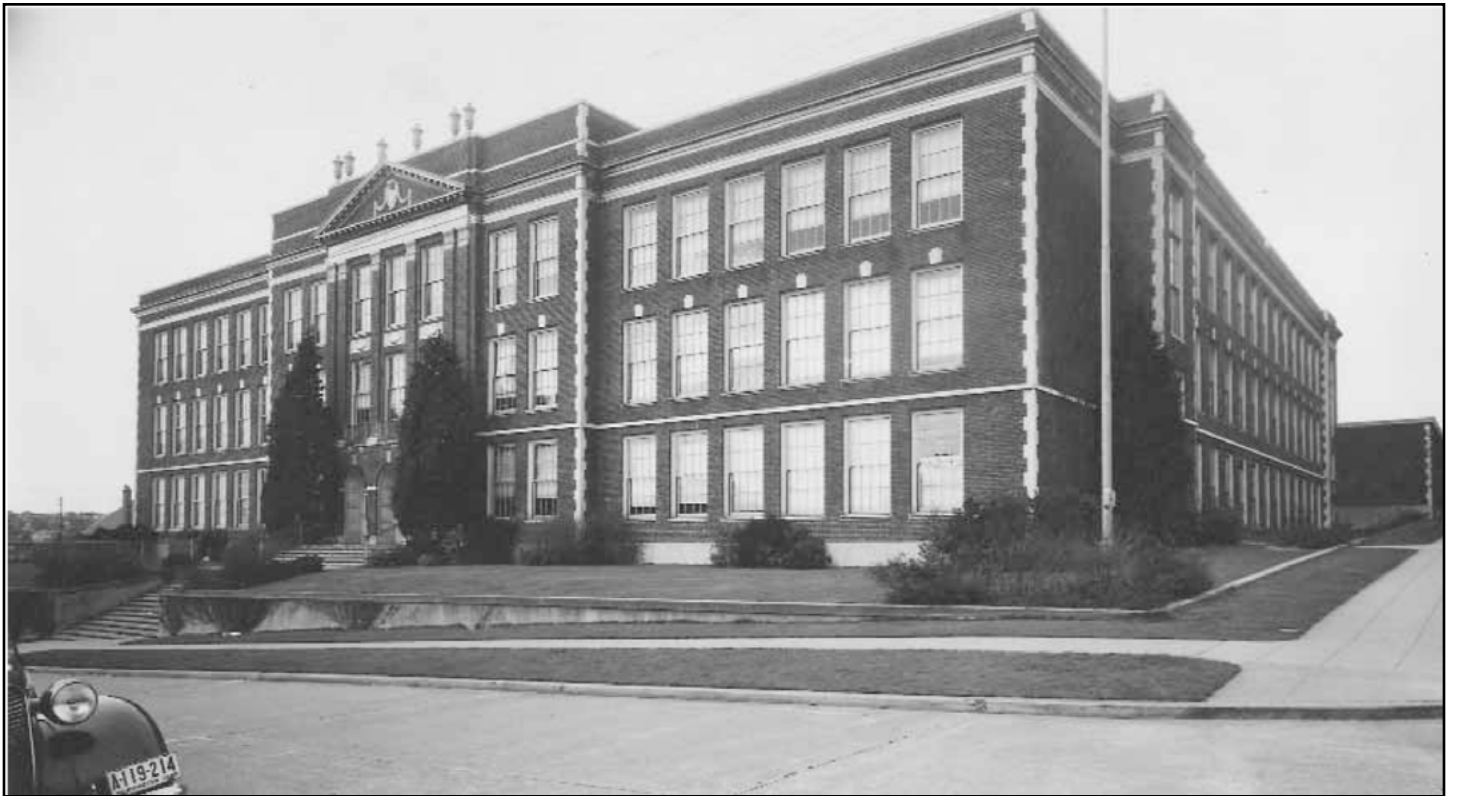
Figure 89. Alexander Hamilton Jr. High School, 1610 N 41st Street (1925, Floyd A. Naramore, altered, Seattle Landmark)
