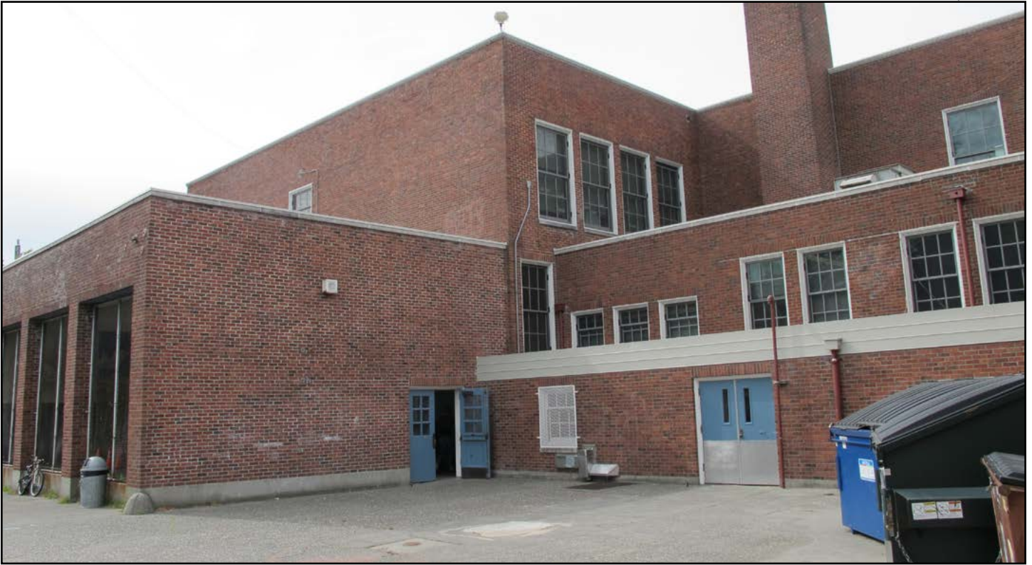
Figure 25. Loyal Heights Elementary School, southern façade, eastern façade of play-court and western wing
