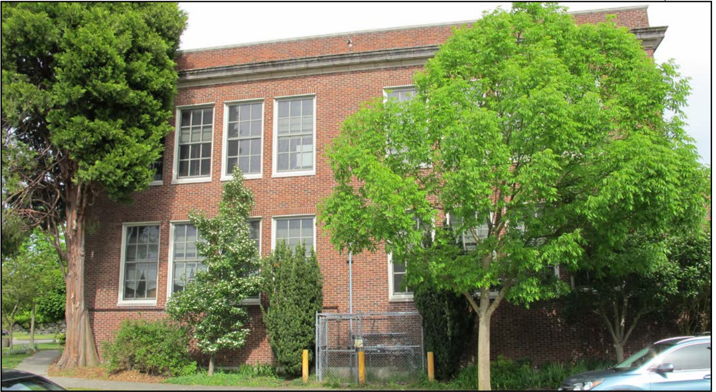
Figure 29. Loyal Heights Elementary School, western façade
