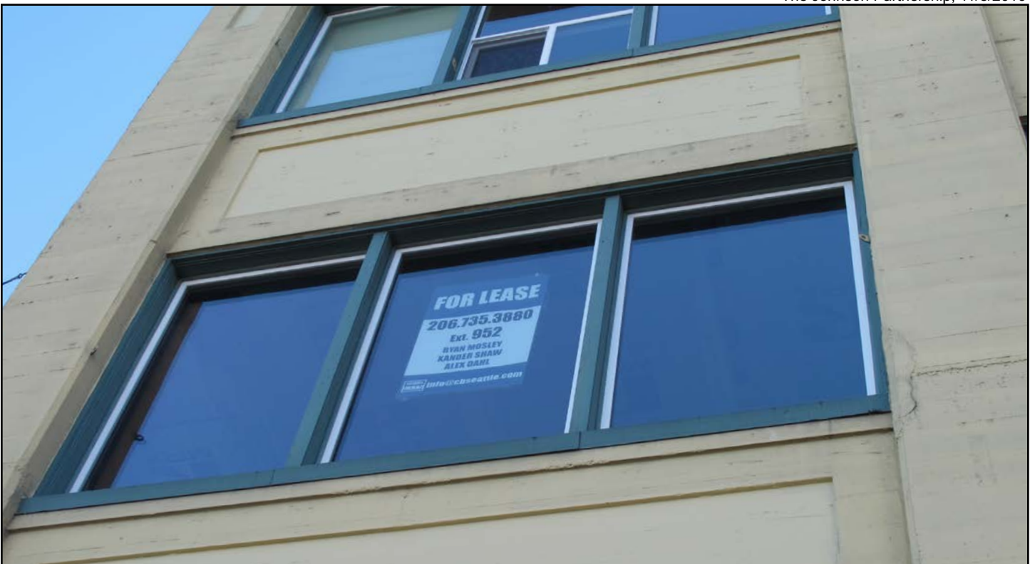
Figure 14. American Meter & Appliance Building, detail of typical windows
