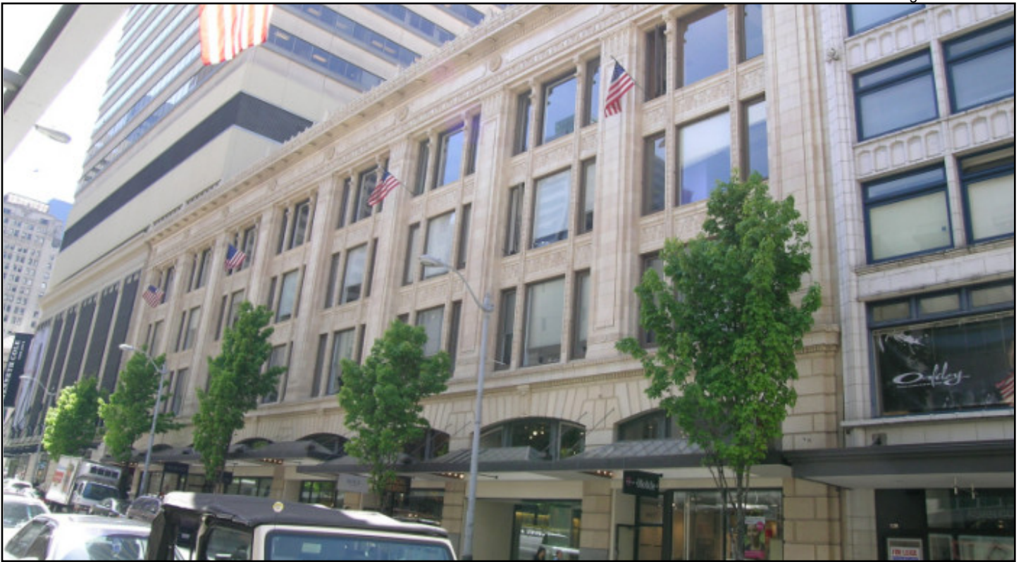
Figure 56. The Decatur Building, 1521 Sixth Avenue (1921-22, Henry W. Bittman, City of Seattle Landmark)
