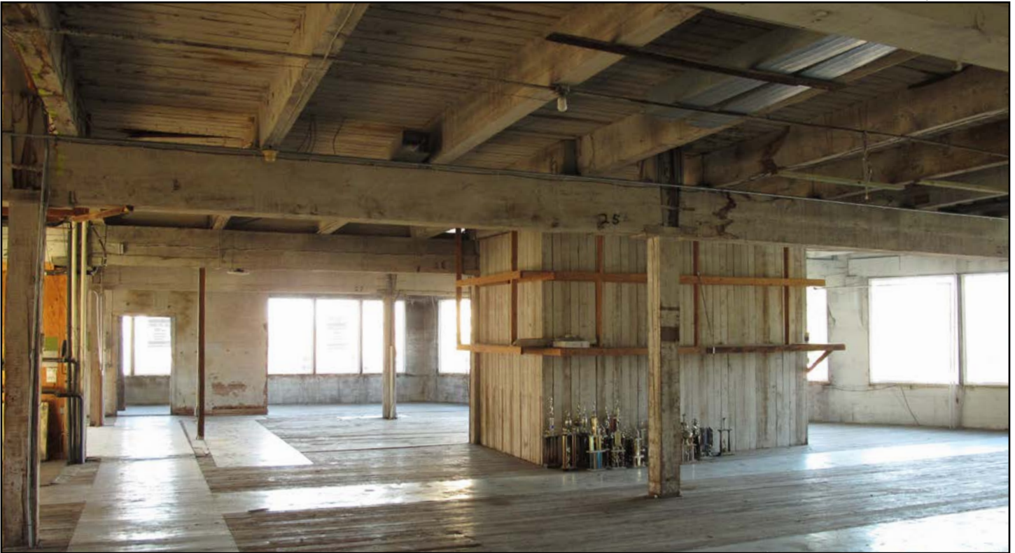
Figure 19. American Meter & Appliance Building, interior at second floor
