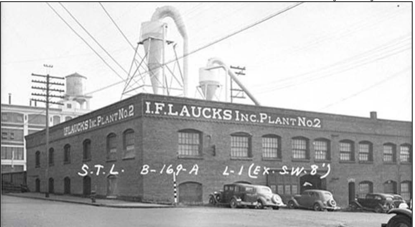
Figure 41. Ainsworth & Dunn Warehouse (1902, City of Seattle Landmark)
