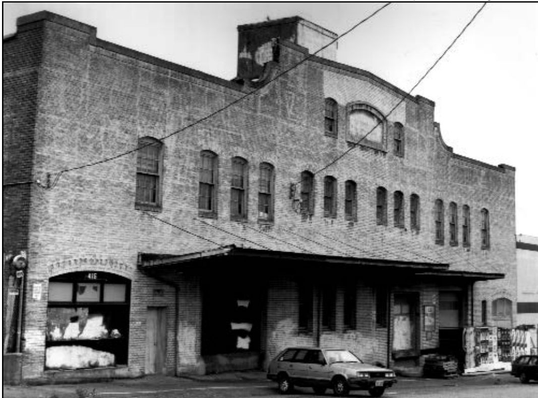
Figure 43. Van Vorst Building (1915, City of Seattle Landmark)
