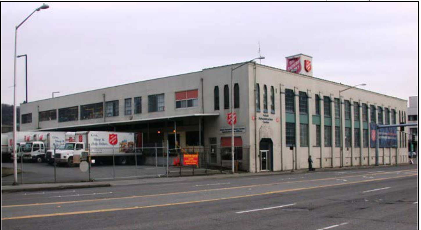
Figure 45. National Grocery Company Warehouse (1930, the Austin Company)
