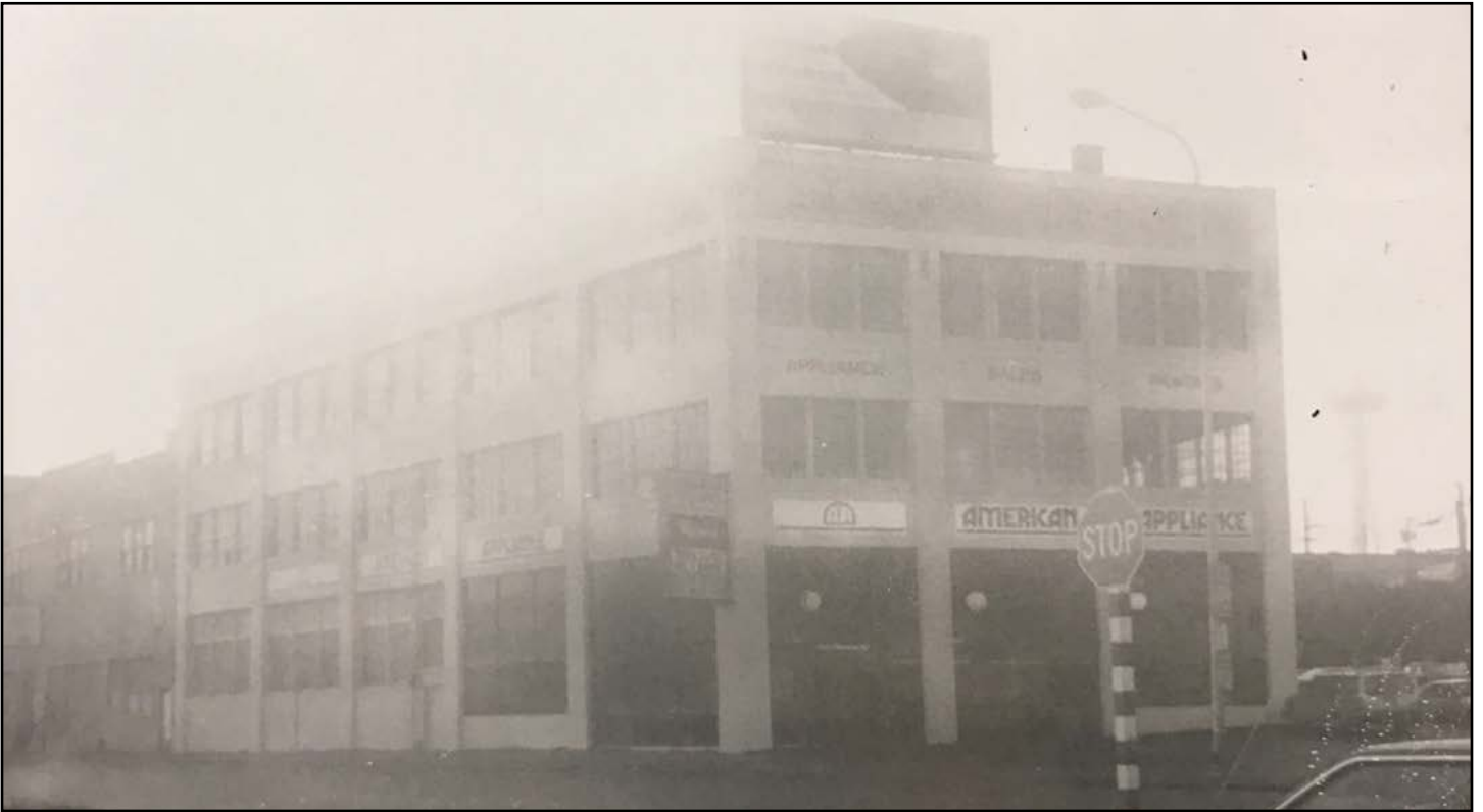
Figure 40. American Meter & Appliance Building, 1974
