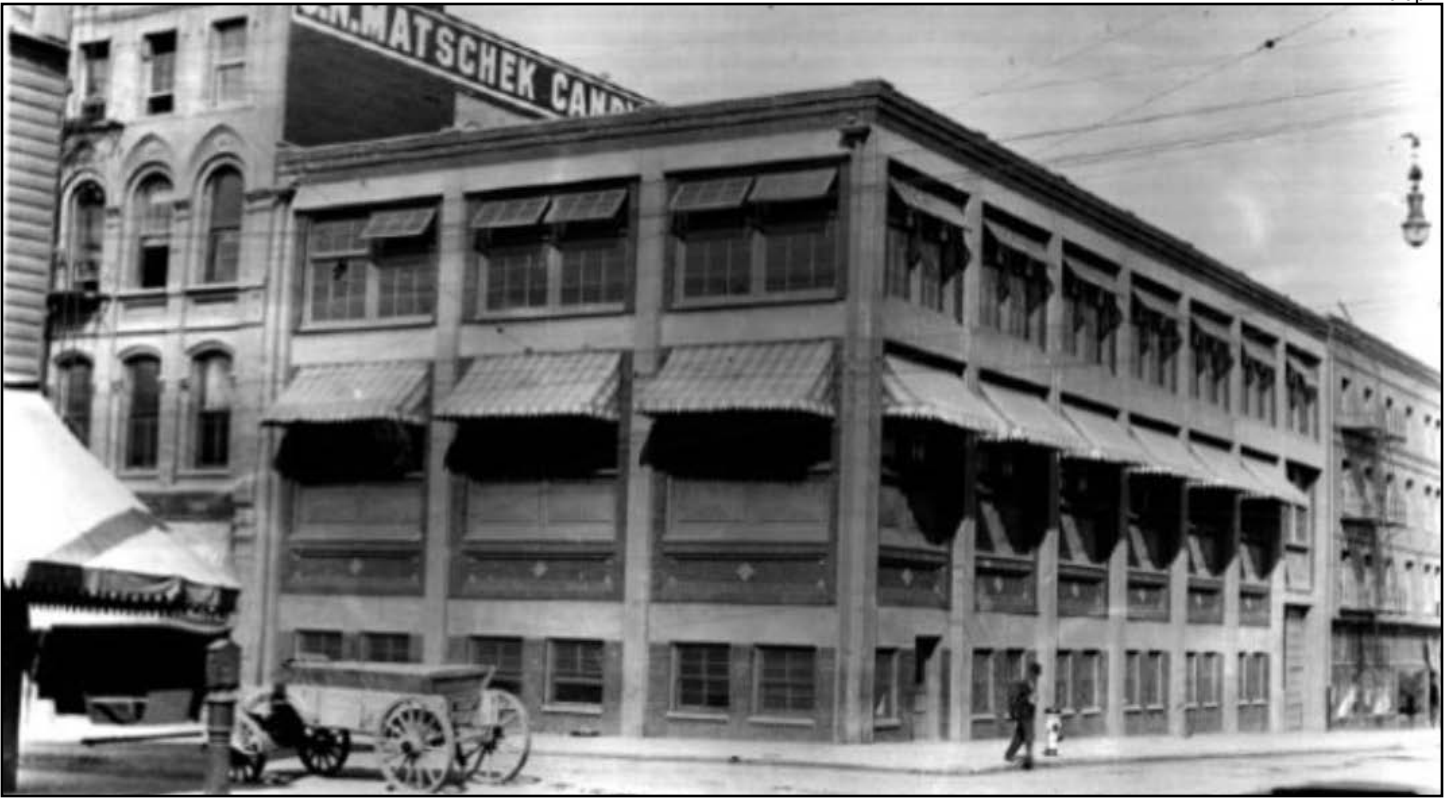
Figure 50. Jefferson Street Substation, 37 SW Jefferson Street, Portland, OR (1909, Hurley-Mason)
