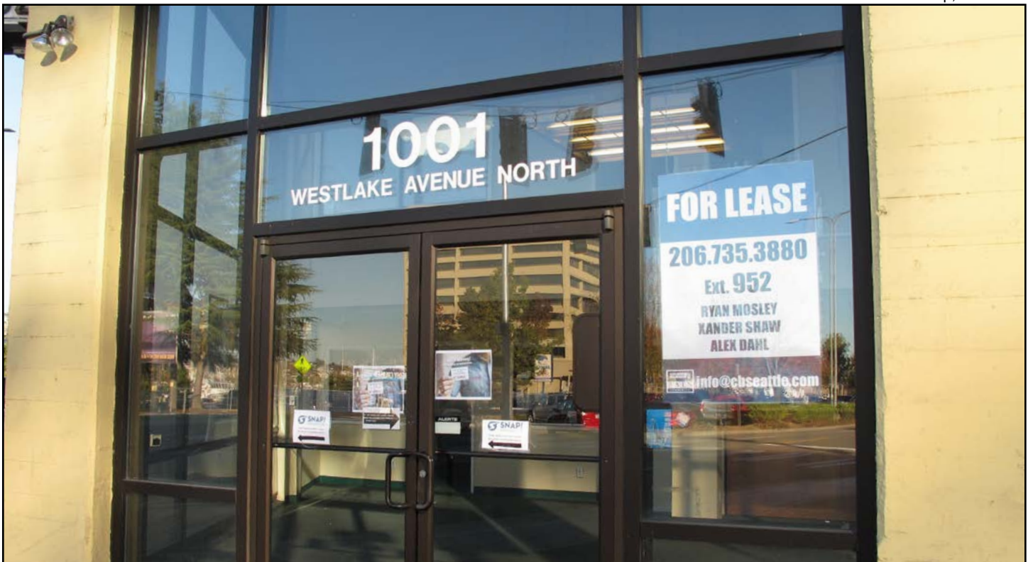
Figure 12. American Meter & Appliance Building, detail of entry door on northern façade
