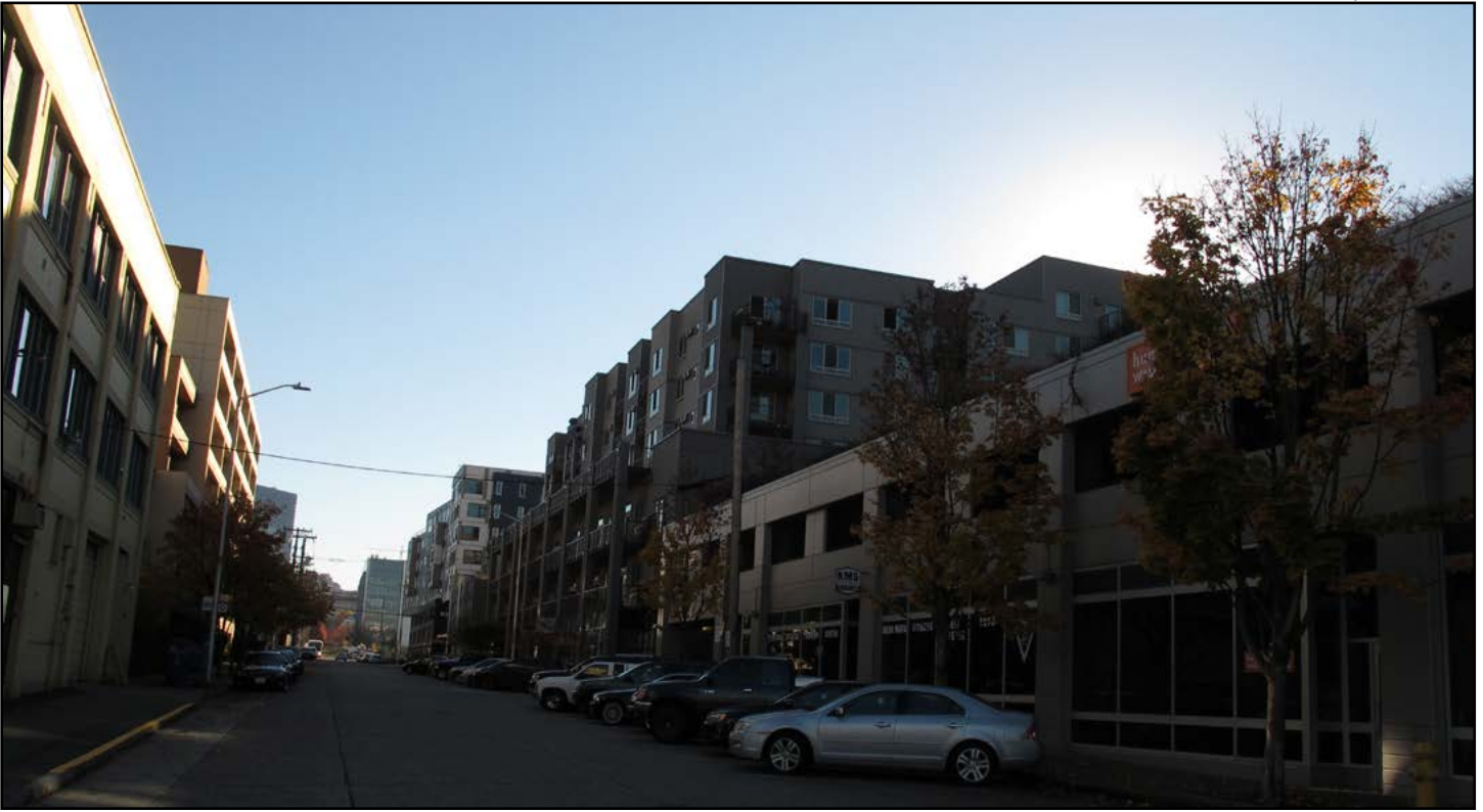
Figure 6. View C—Viewing south on Ninth Avenue N
