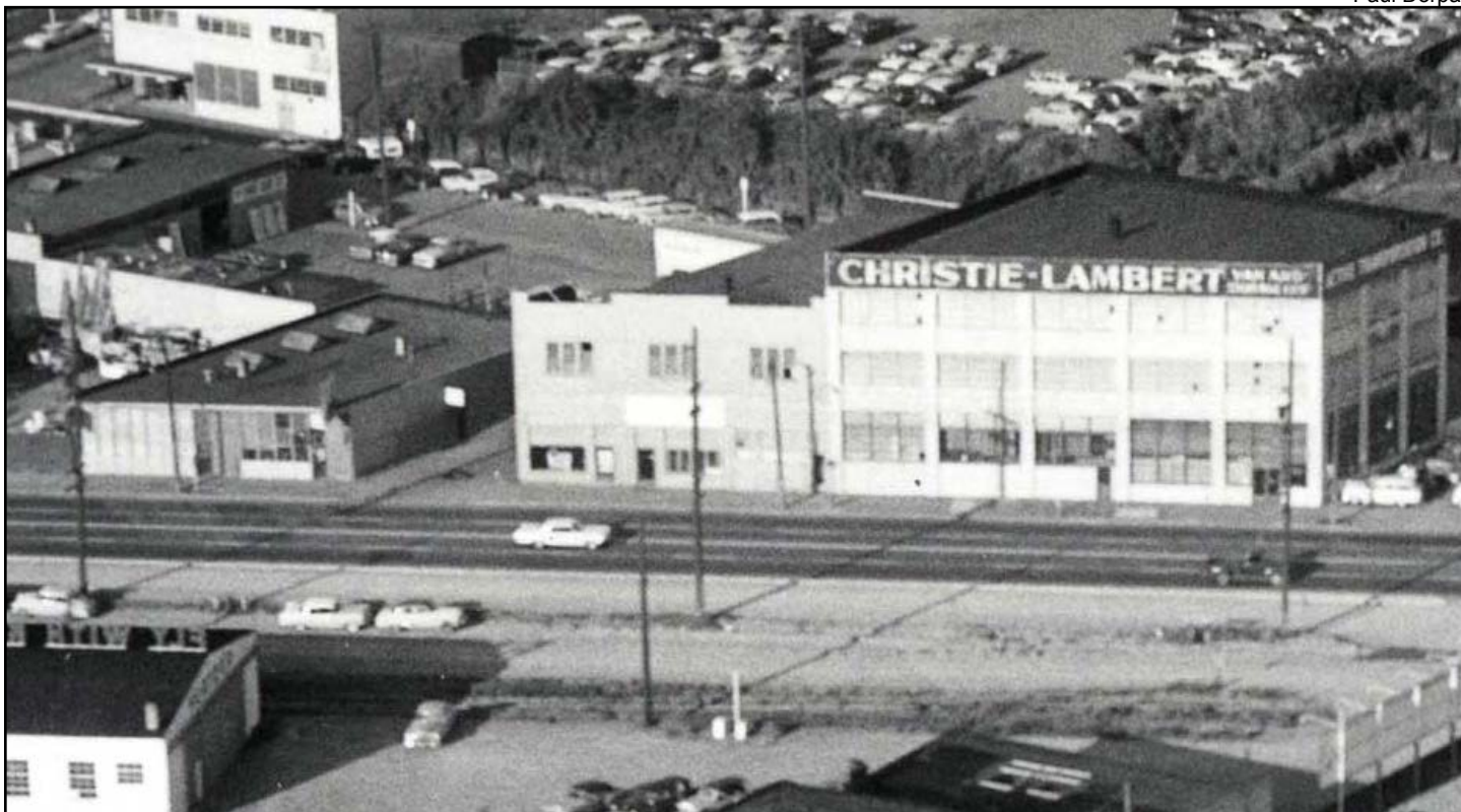
Figure 38. Christie-Lambert Building, now called American Meter & Appliance, ca. 1957
