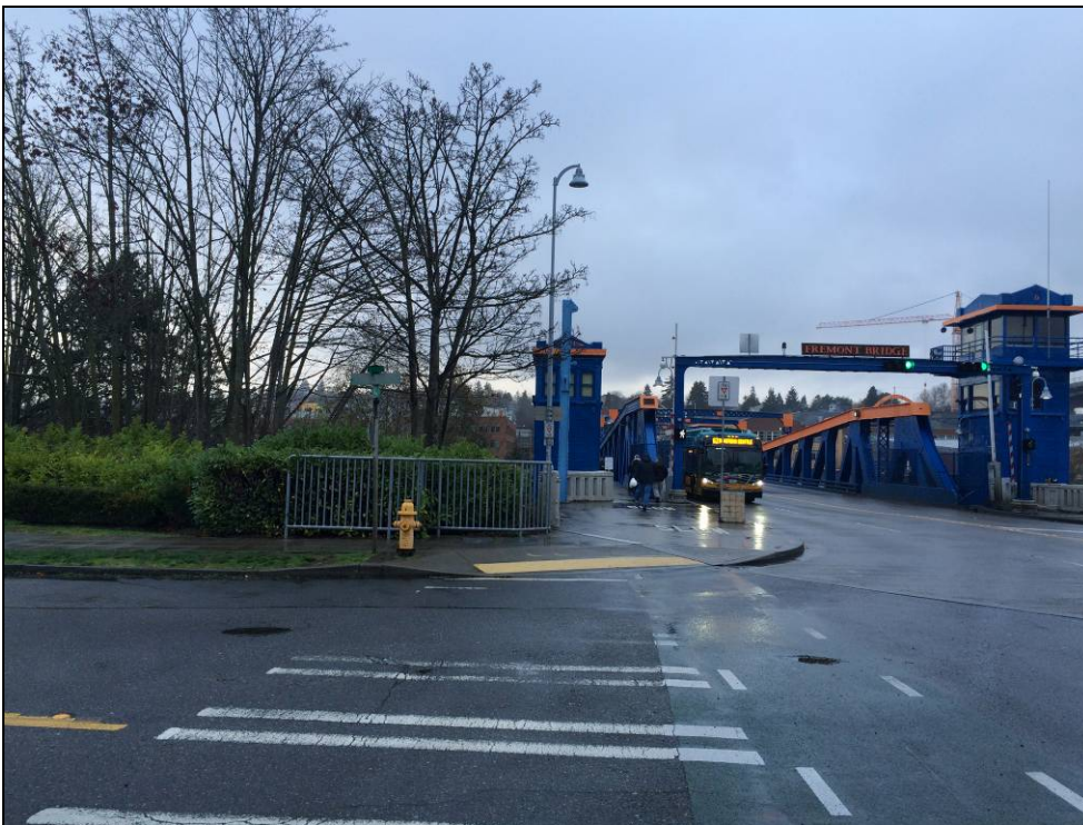
Figure 15. Below, looking north across the Fremont Bridge at the intersection of 4 th Avenue N and Florentia Street.
