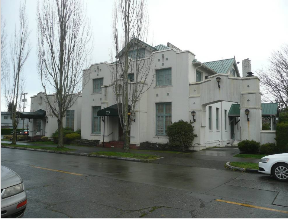
Figure 24. Above, looking northwest at the primary south and secondary east facades.
