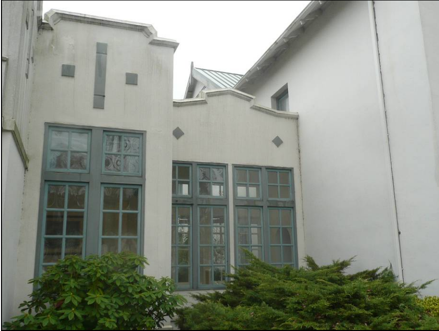
Figure 28. Above, looking north at the link between the new section (left) and portion of the original west facade (right).
