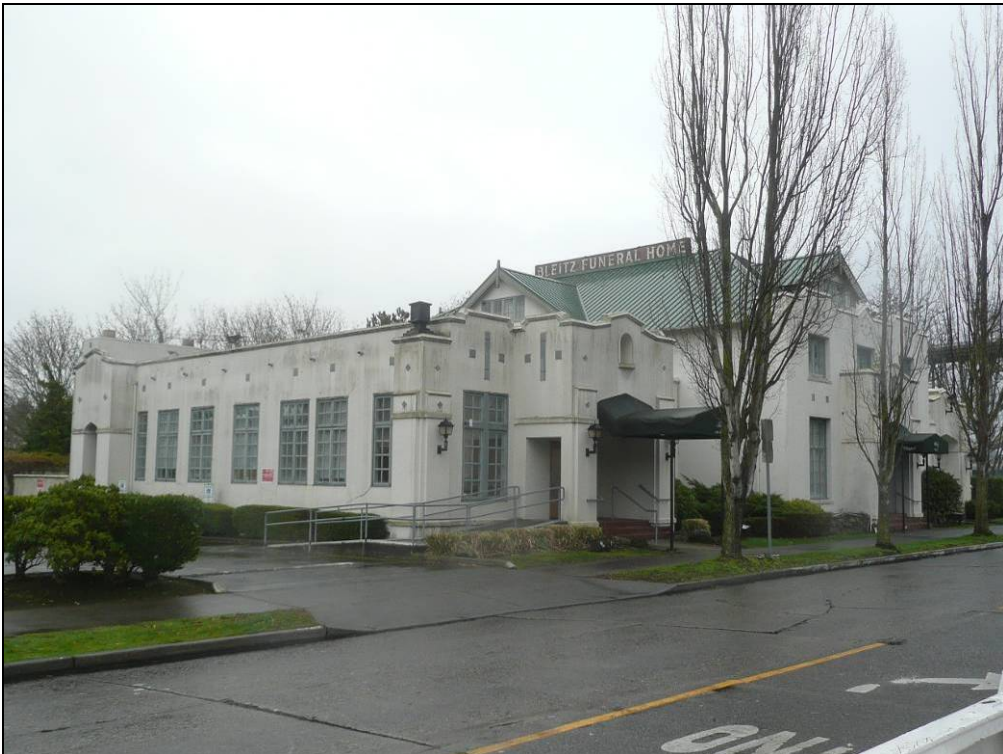
Figure 27. Below, looking northeast at 1988 office addition (left) and the original building (right).
