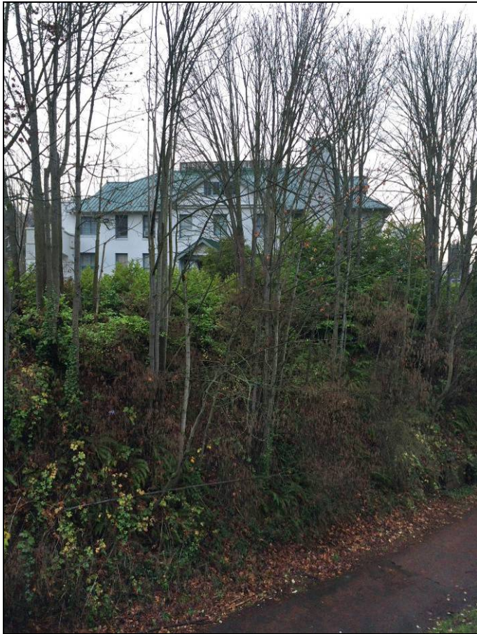
Figure 11. Left, looking west at the building with the South Ship Canal Trail visible in the foreground.
