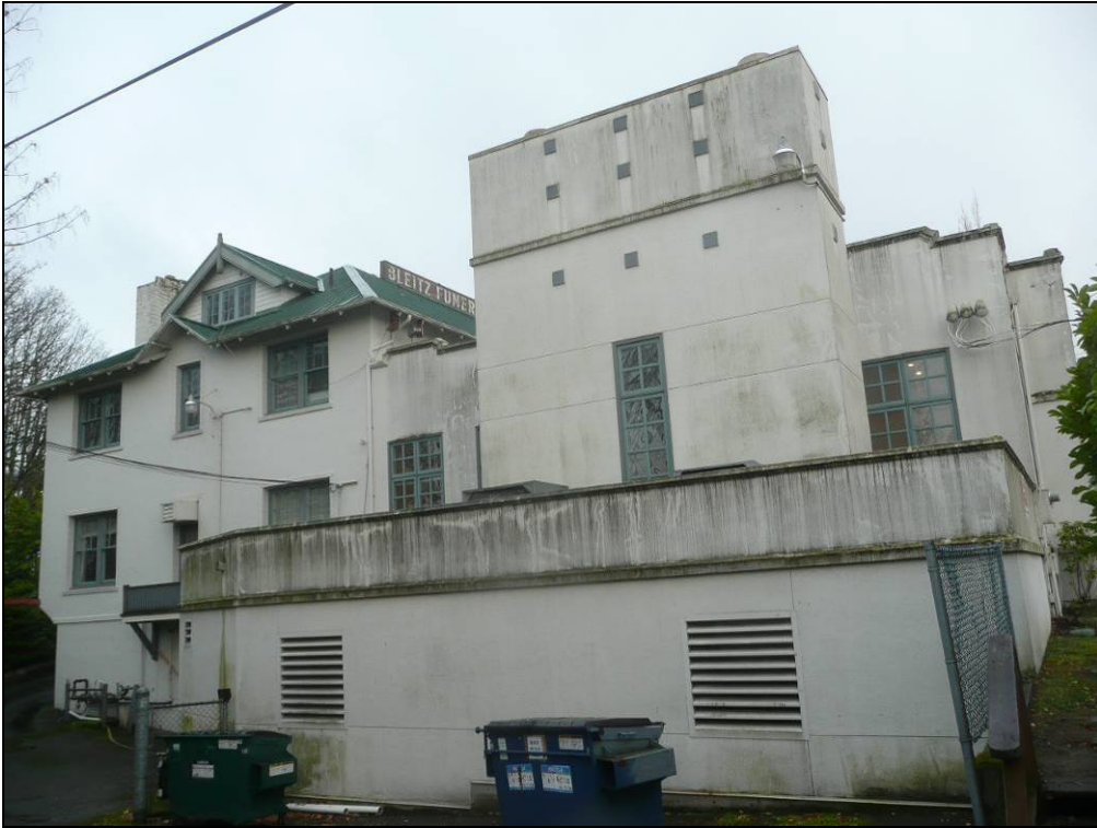
Figure 26. Above, looking generally southeast at the back (north facades) with 1988 west addition to the right and 1991 crematory addition in the foreground. The original building (left to the east) is distinguished from these additions by its massing, roof shape, materials, and details.
