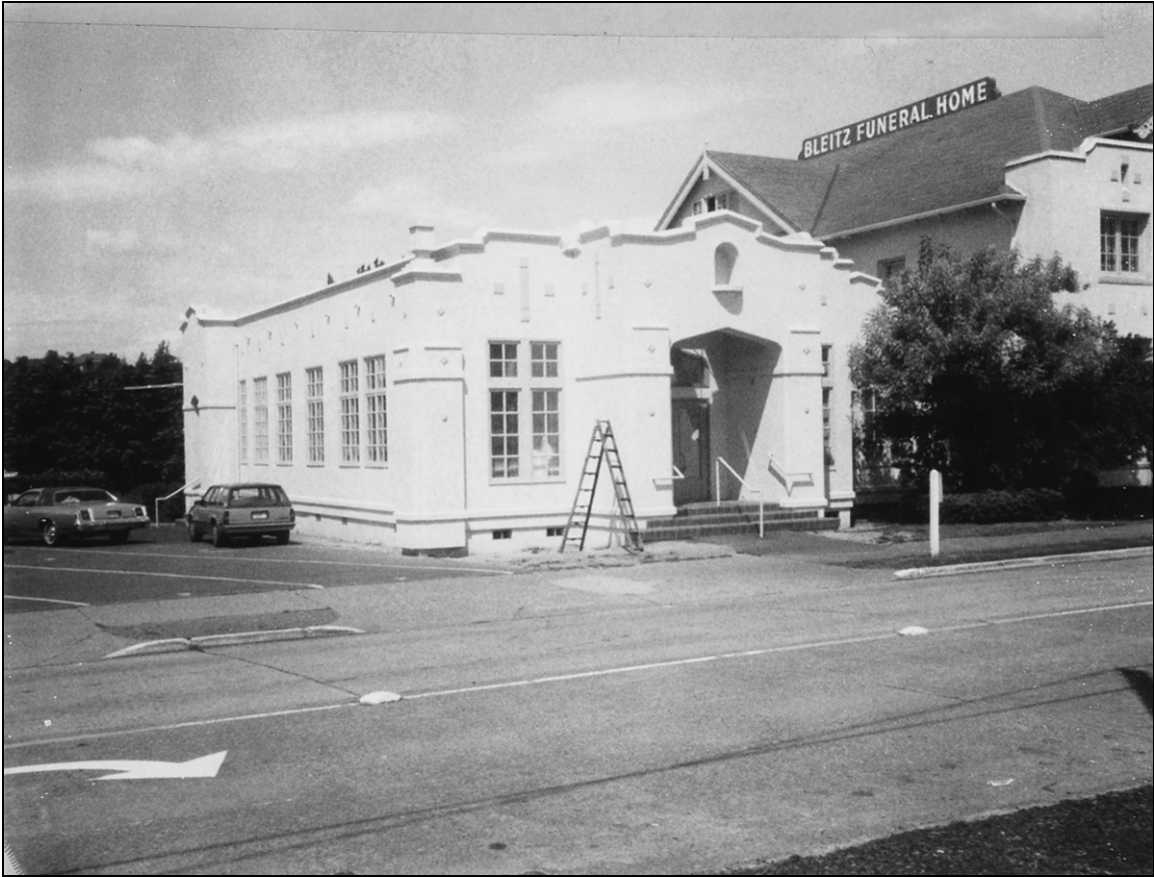
Figure 22. Above, a King Co. Tax Assessor's photographs of the 1989 addition under construction with the original building in the background right (Puget Sound Regional Archives).
