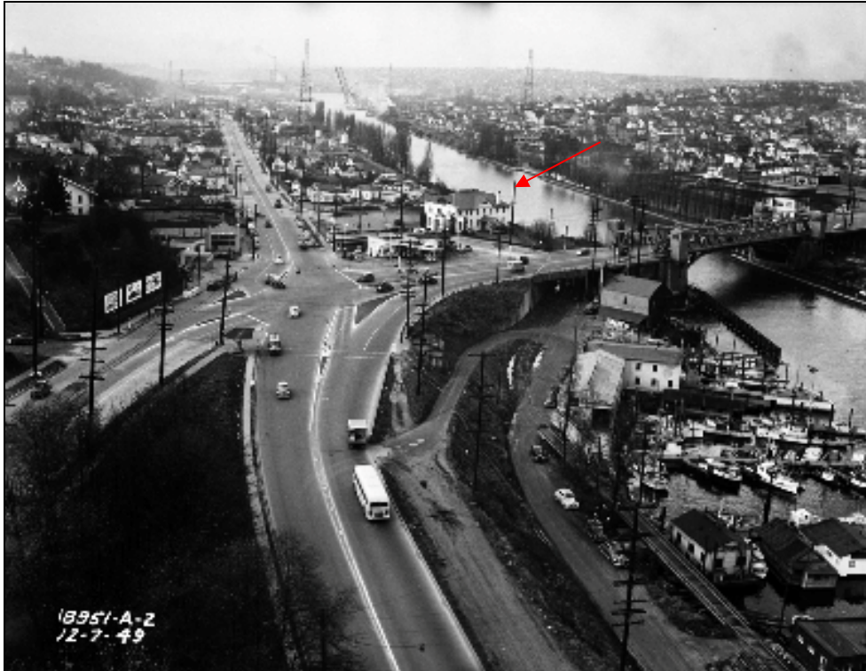
Figure 9. Above, looking northwest, in 1949. The subject building is noted by a red arrow (SMA image 54371).
