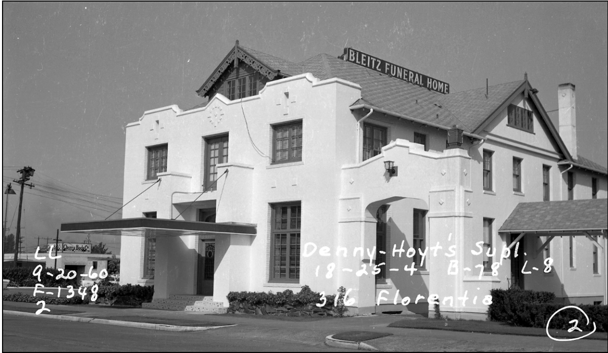
Figure 20. Above, a 1960 King Co. Tax Assessor's photograph. By this date the half-timber treatment in the side gable end had been painted, and a new Modern style marquee added to what was then the main entry.
