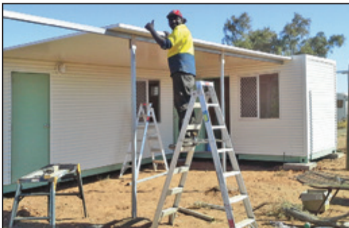
Andrew Alice works on a container home at Urrermerne.
