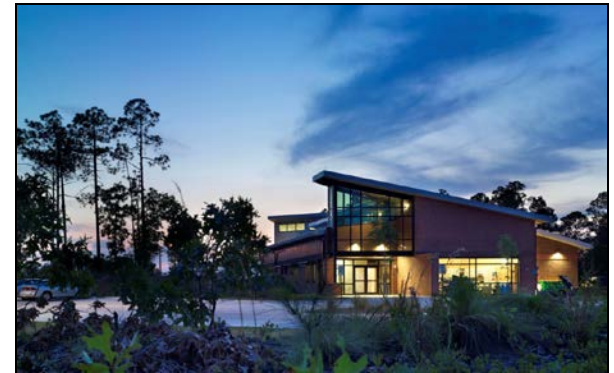
Fort Bragg LEED Platinum Community Emergency Services Station Photo credit: USACE Savannah District
