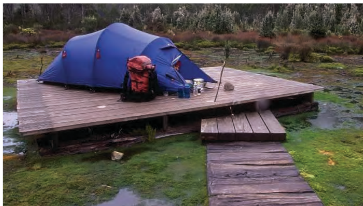
Example of a tent platforms along the Overland Track in Tasmania. The use of elevated tent platforms and raised boardwalks has become the recognised means to provide a quality camping experience, while protecting the surrounding, sensitive environment
