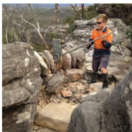
Construction of a stone stairway leading to Mount Rosea demonstrating high quality craftsmanship, use of local stone and avoiding the need for handrails or balustrades through good trail alignment.
