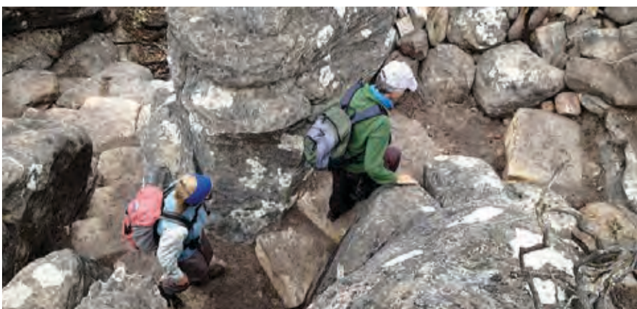
Construction of a stone stairway leading to Mount Rosea demonstrating high quality craftsmanship, use of local stone and avoiding the need for handrails or balustrades through good trail alignment.
