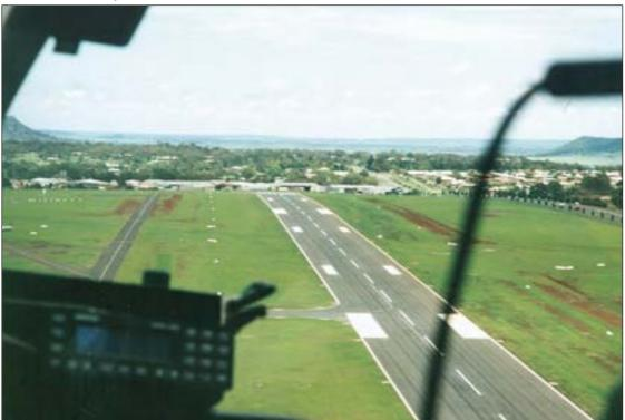
Examination of Toowoomba City Council engineering diagrams indicated that for the first 170 m of runway 29 there was an upward slope in excess of 1.25 per cent. This slope gradually reduced until the peak of the runway, which occurred at a point 780 m from the runway 29 threshold. The runway then sloped downward to the west at a gradient of about 1.5 per cent for the last 40 m. The effect of the upward slope was to increase the take-off run of an aircraft (see Section 1.20.6).
