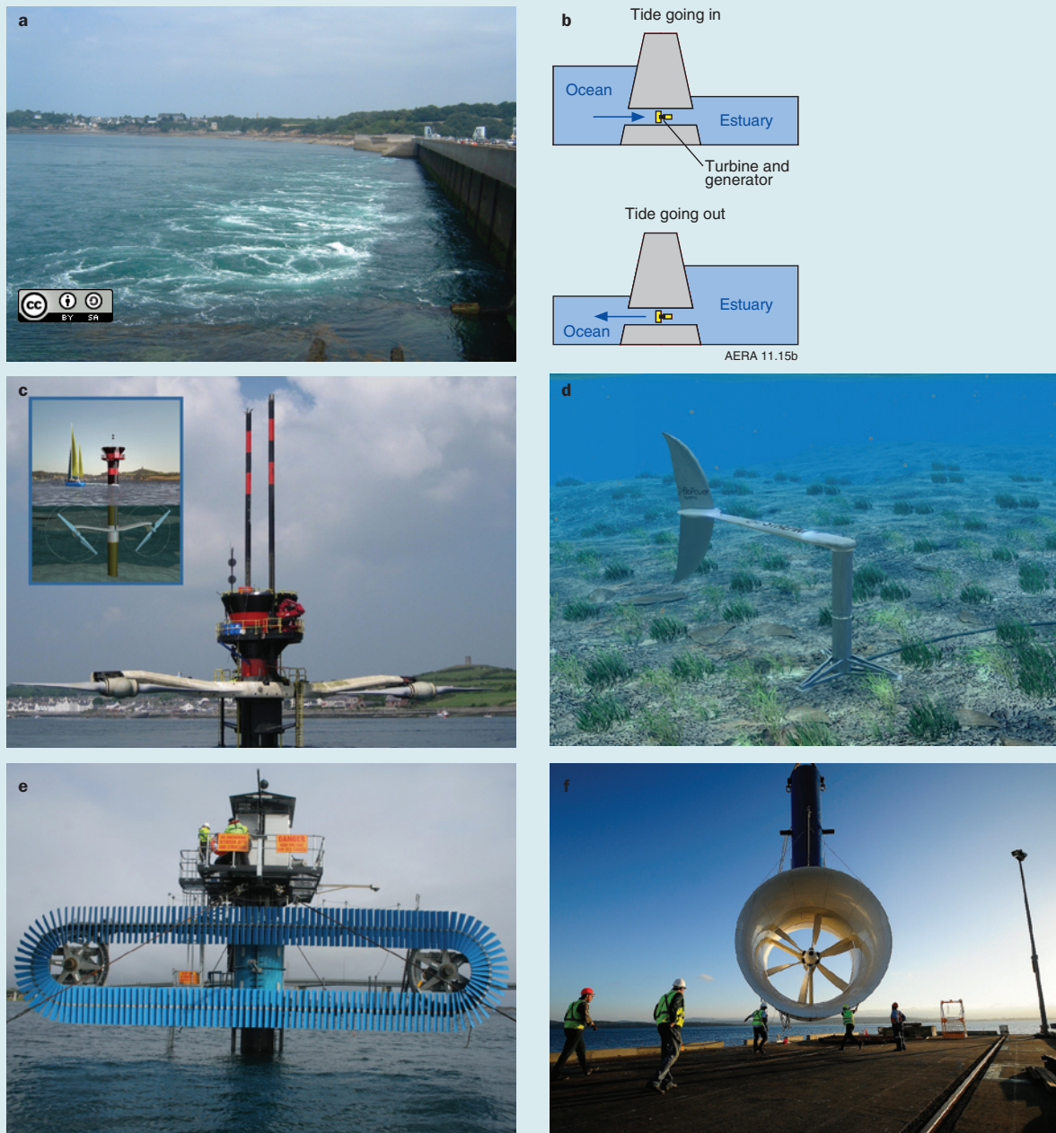
Figure 11.15 Examples of different types of tidal energy converters. (a) La Rance River estuary tidal barrage (b) Schematic showing the water levels either side of a barrage during power generation (c) Sea Generation Ltd's SeaGen turbine with blades elevated for servicing (d) BioPower System's bioStream turbine (e) and (f) Atlantis Resources Corporation's Nereus and Solon turbines, respectively
