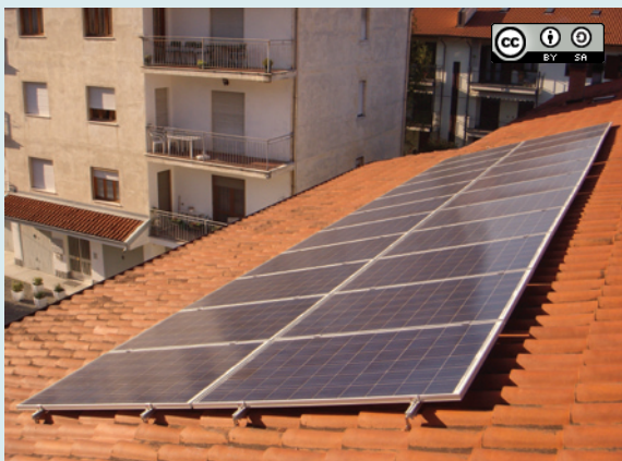
Figure 10.25 (a) Example of a rooftop PV system. (b) A schematic concentrating PV system, where a large number of mirrors focus sunlight onto central PV receivers
