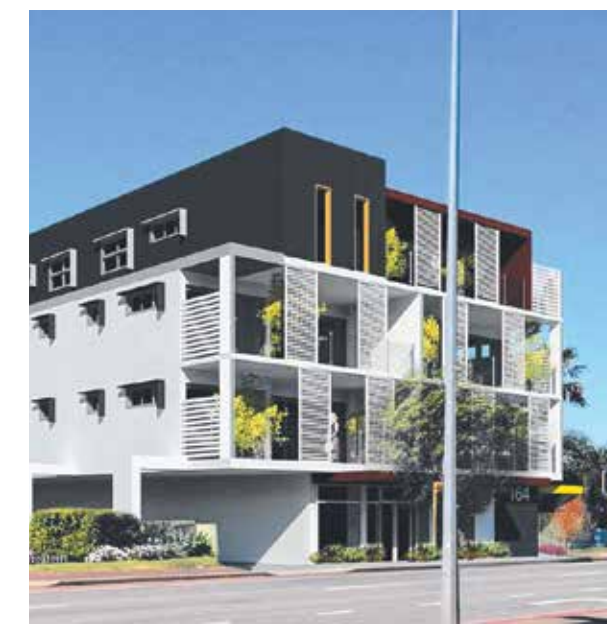
Booragoon units are the quickest-selling in Perth. Picture shows artist's impression of 164 Riseley St, Salt Property Group, Harden Jones Architects.
