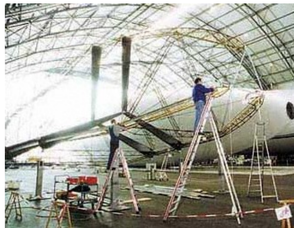
Fig. 22. Triangular frames and longerons in Zeppelin NT
