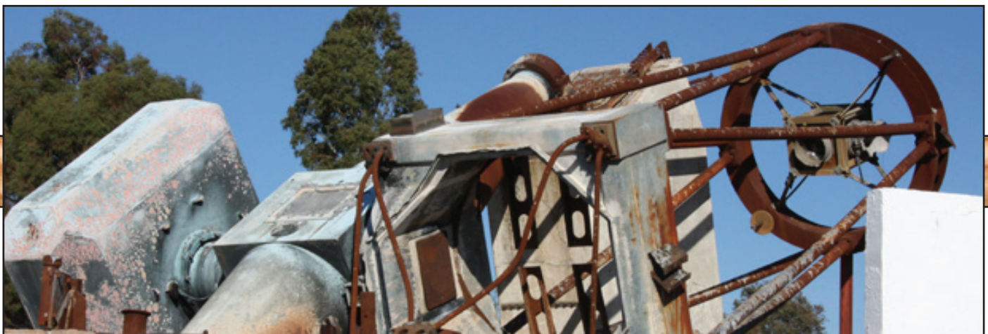
The damaged GMT at Mt. Stromlo. Note the absence of the dome.
