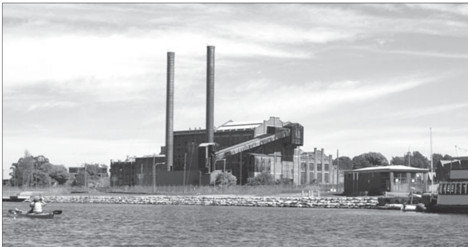
The vast, brooding White Bay Power Station, which dominates White Bay and Rozelle Bay, is disused, but has wonderful potential for other purposes.
