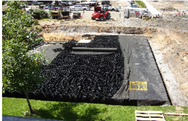
The construction of 170,000 litre underground water tanks at Monash University, NSW, as downloaded from the Monash University website at http://www.monash.edu.au
