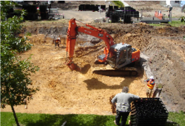
The construction of 170,000 litre underground water tanks at Monash University, NSW, as downloaded from the Monash University website at http://www.monash.edu.au
