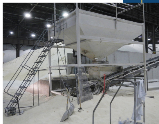
The sugar hopper where a temporary worker was buried alive, part of a story on temp worker safety ProPublica published with Univision.
