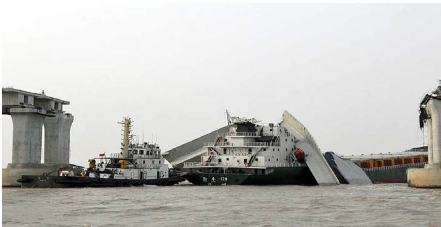
March 27, 2008: A 60-meter section of Jintang Bridge fell onto a cargo ship near the eastern port city of Ningbo, east of China's Zhejiang province. Photo credit: AP Images
