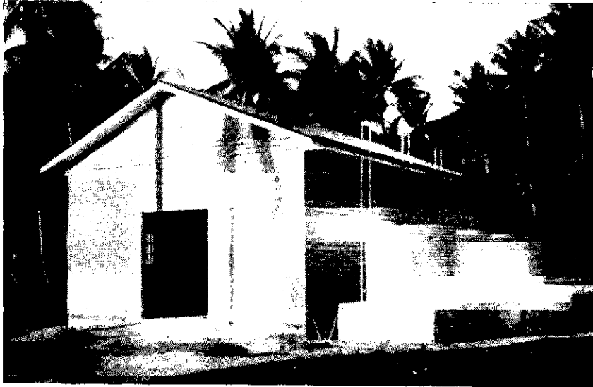
Power House. Electricity Supply.
