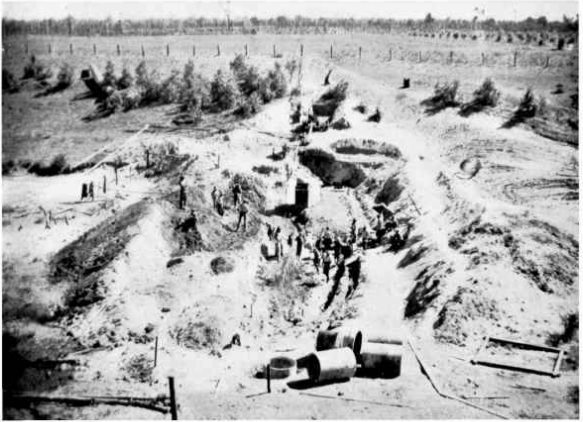
Successfully Tapping Underground Water Supplies, Mimosa Creek, Woorabinda.
