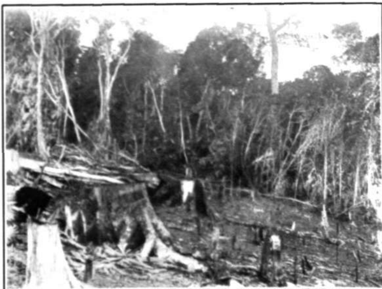
Hull River Settlement—Portion of Clearing.
