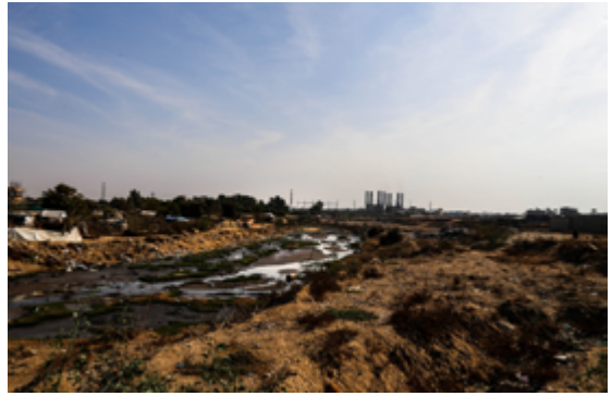
Sewage in Wadi Gaza, with the power plant in the background. Wastewater contaminates drinking water.
