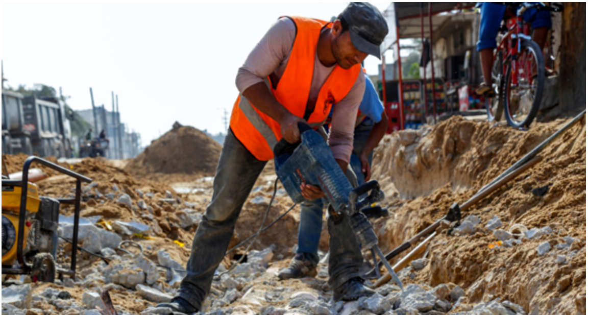
Maintenance of water infrastructure in Gaza. A third of the water is lost due to defective and damaged pipes.
