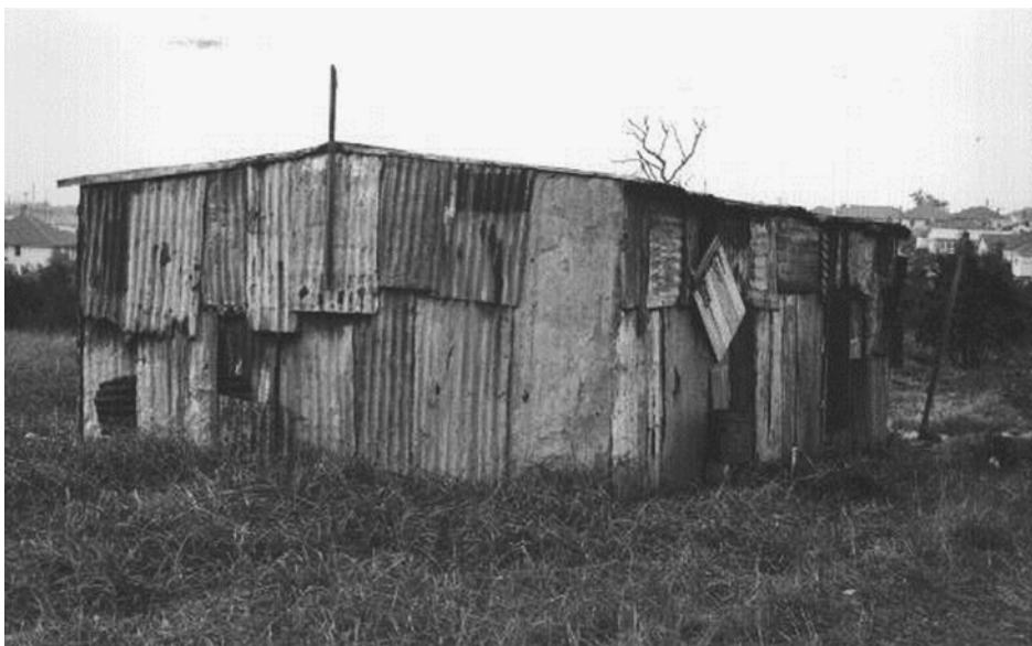
Figure 1: A Platt's Estate residence, May 1960 (photograph courtesy of Ronald John Morisson)
