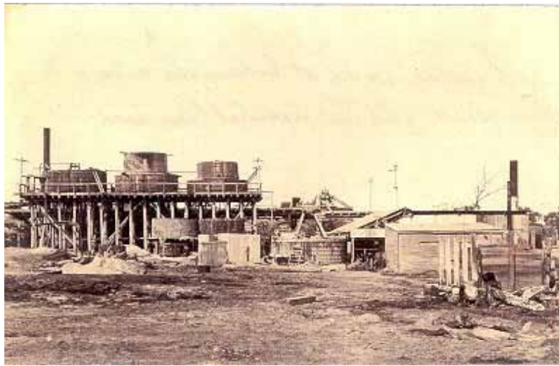
Figure 45 Cyaniding Plant Gold mine at Bodangora
