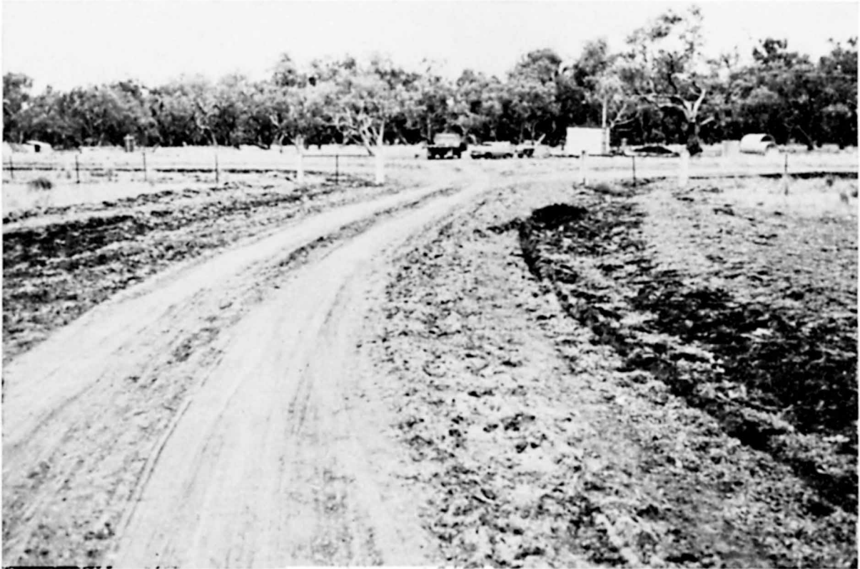
This photo shows the access road to the fenced-off Tulladunna camp, with the washing facilities under construction.
