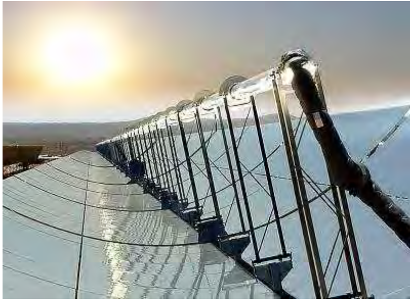
Figure 11: Parabolic trough (north-south axis view)
