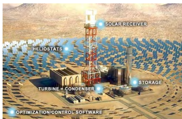
Figure 8: Brightsource Energy’s LPT 550 system—the Ivanpah Station
