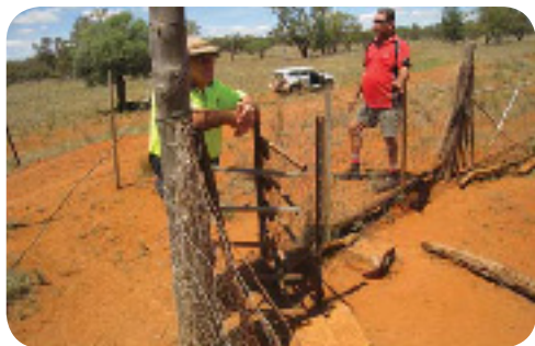
Workers replacing old fencing on Mawonga.
