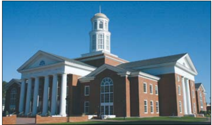
The new Paul and Rosemary Tribble Library on the Christopher Newport University Campus in Virginia.
