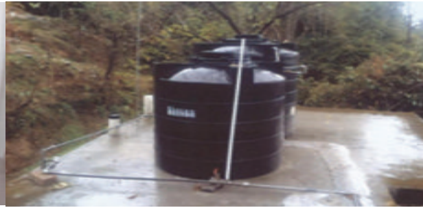
Thangtong Lughar water project completion of alleviated the drinking water scarcity.
