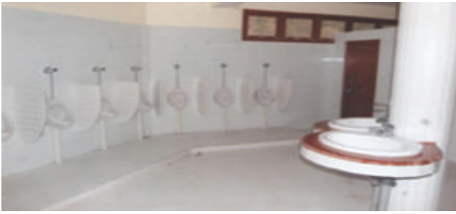
Public toilet renovation was completed in Bir Tibetan Settlement on 17 February 2013.
