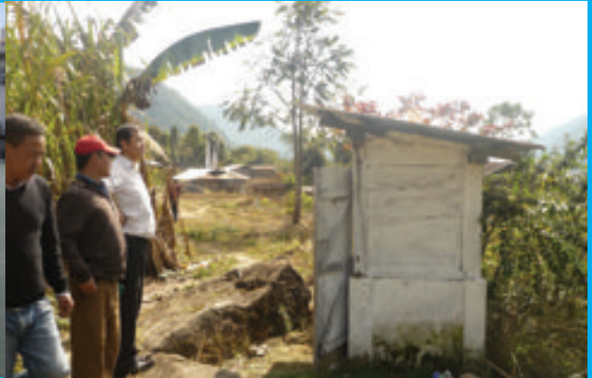
Inspecting the existing toilet facilities in the remote Tuting settlement
