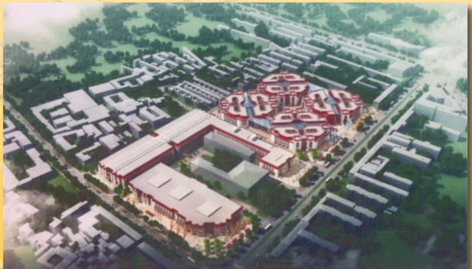
A display image of the Barkhor Shopping Mall, currently under construction
